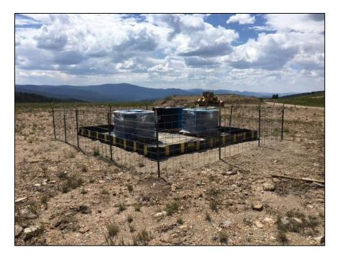
Photograph 6: Chemical storage area with secondary containment and fencing
