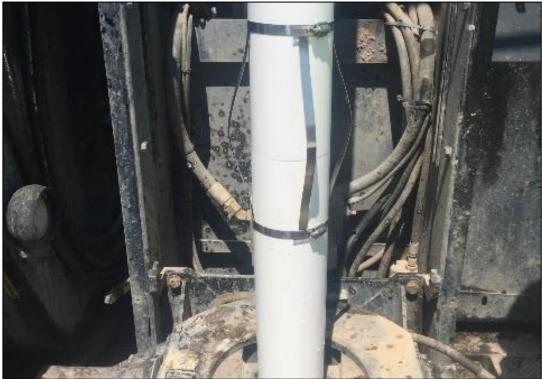
Photograph 23: Indian Rock Dump piezometer installation showing centralizer on RD-07
