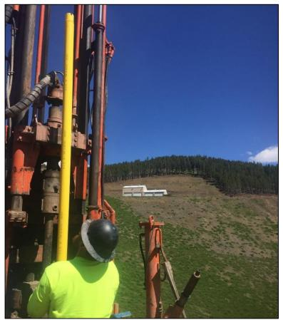
Photograph 26: Installing slope inclinometer casing at IN1
