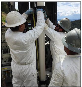
Photograph 18: Primary grout cone placed at 90 feet below ground surface in piezometer P-14
