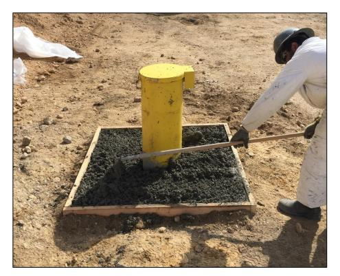
Photograph 20: Concrete pad being constructed at piezometer P-13
