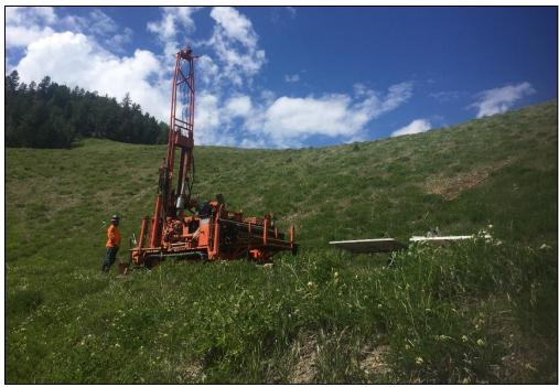
Photograph 25: Drilling IN2 with combination of ODEX® down-hole air hammer system and hollowstem auger
