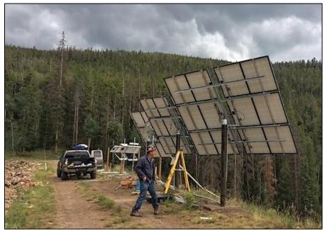
Photograph 31: Solar panels installed on the sediment control pond embankment
