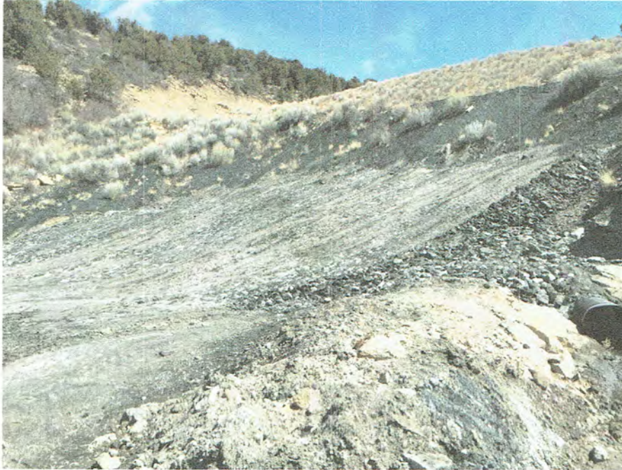
Pic. 3 – New material installed at base of embankment/waste pile.
