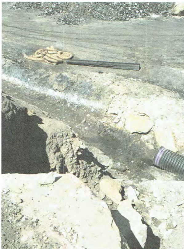
Pic. 4 – Grading improved at outlet of under drain from Reach 10 ditch.
