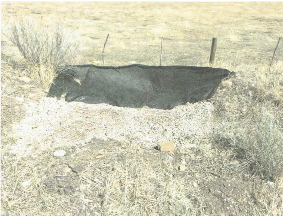
Pic. 4 – Sediment trap along east side of driveway has been repaired.
