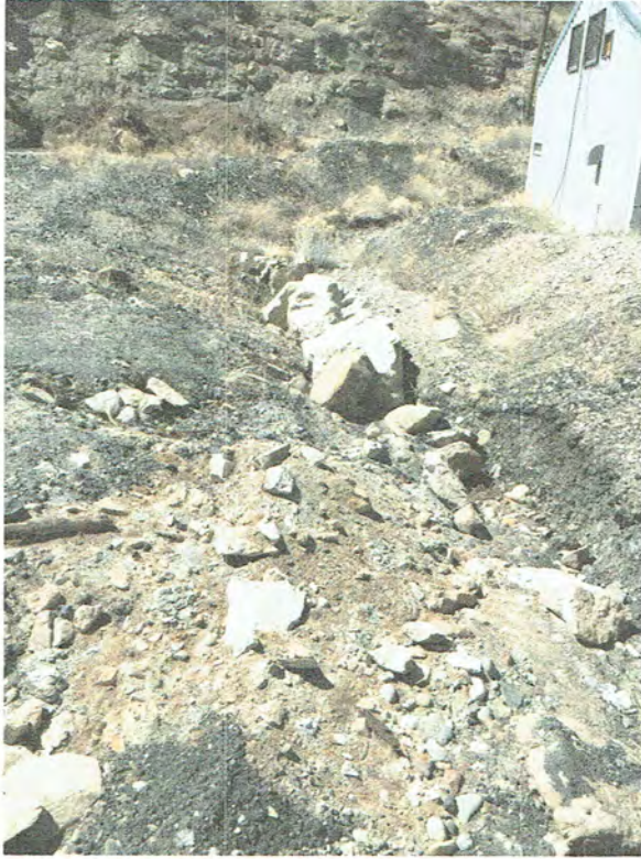
Pic. 3 – New riprap in ditch to west pond.
