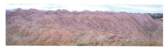
This photograph (looking northwest) shows the north brick stockpile that has been removed and placed into the pit on the left side of the picture. On the right side of the picture is the area that has been backfilled.
