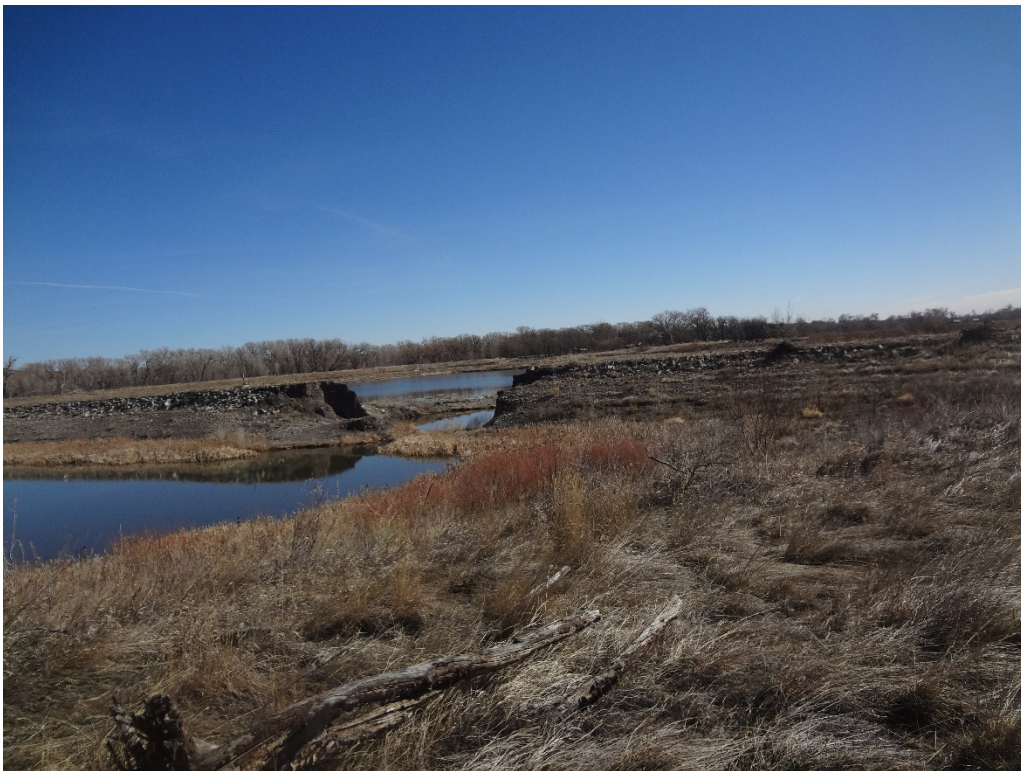
View of the south slurry wall breach in Lake 4 looking northeast
