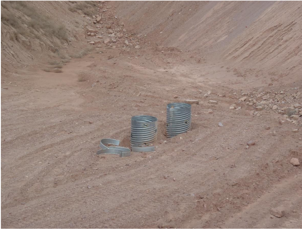
Photo 6. Stormwater pond risers.
