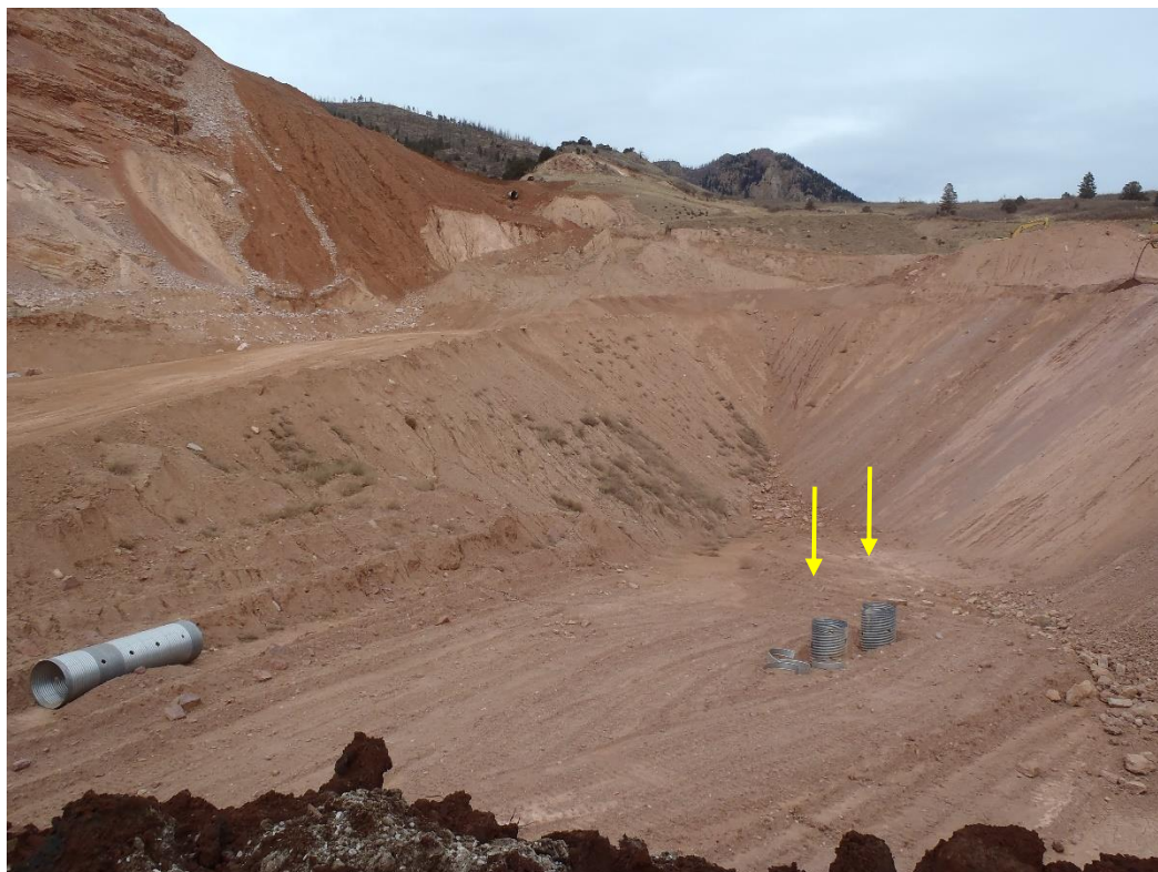
Photo 3. Riser pipes in stormwater detention pond (looking NNW).
