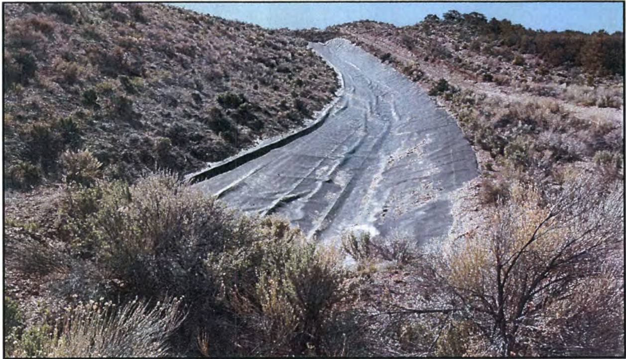
Photo 29 Looking southeast up the left downstream groin from the access road. Note the absence of significant sediment deposits on the liner along the groin.
