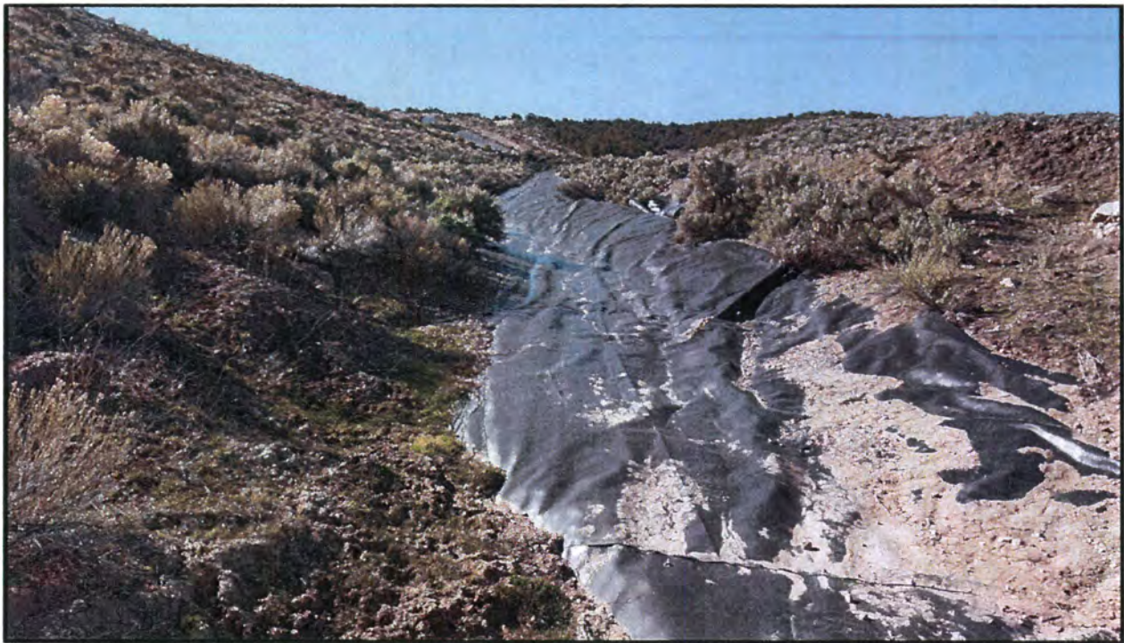
Photo 26 Looking southeast from the bottom of the left downstream groin. Note the absence of significant sediment deposits on the liner along the groin.
