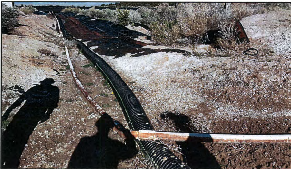
Photo 13 Looking west over toe drain outfall pipe toward seepage collection pond. Note that there is almost no water flowing along the pipe in the lined channel.
