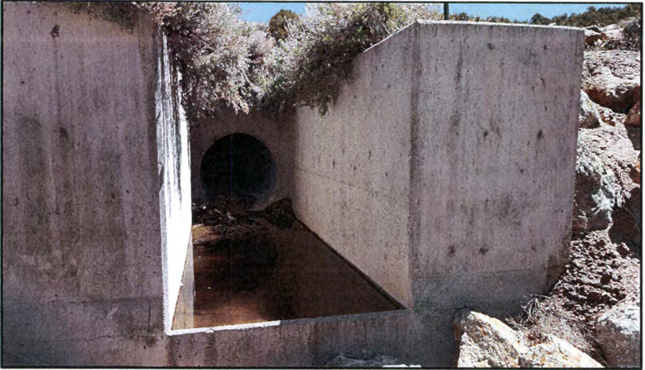
Photo 19 Looking east at the drop structure outlet. Note minor sediment buildup and bushy vegetation beginning to take root.
