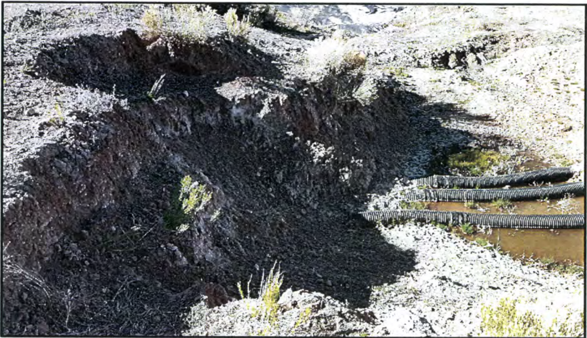
Photo 11 Looking south over toe drain discharge pipes. Note shallow standing water around pipes, but no seepage in the embankment above the pipes.
