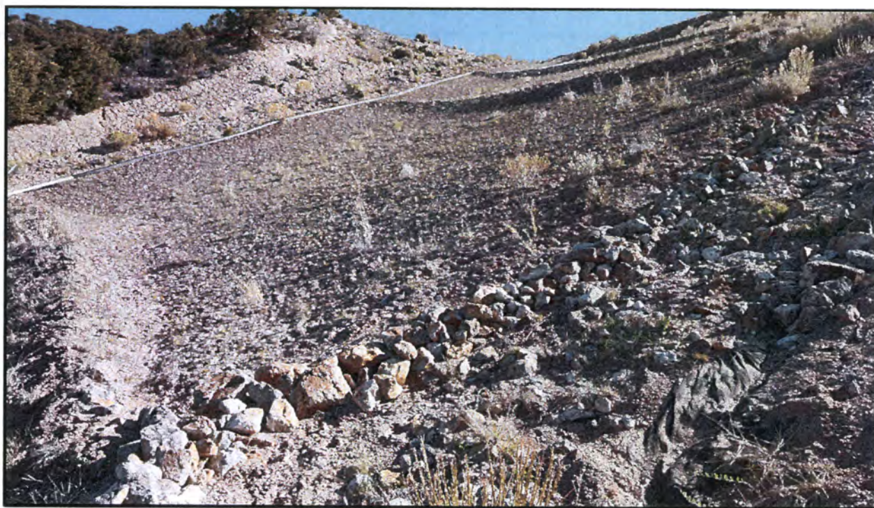
Photo 24 Looking northeast over recently repaired and re-seeded area at the right downstream groin. Note the emergence of new vegetation in the area, and minor erosion of the rock-lined drainage path exposing the filter fabric beneath.
