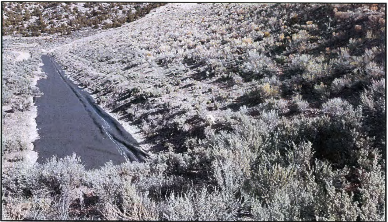
Photo 28 Looking northwest across the left downstream groin and lower downstream face from the access road. Note the absence of significant sediment deposits on the liner along the groin.
