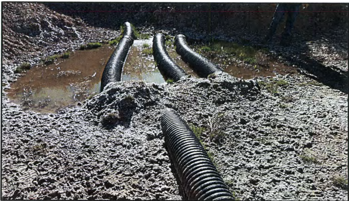
Photo 12 Looking east over toe drain discharge pipes. Note 3 pipes draining to a manifold, then to a single outfall pipe.
