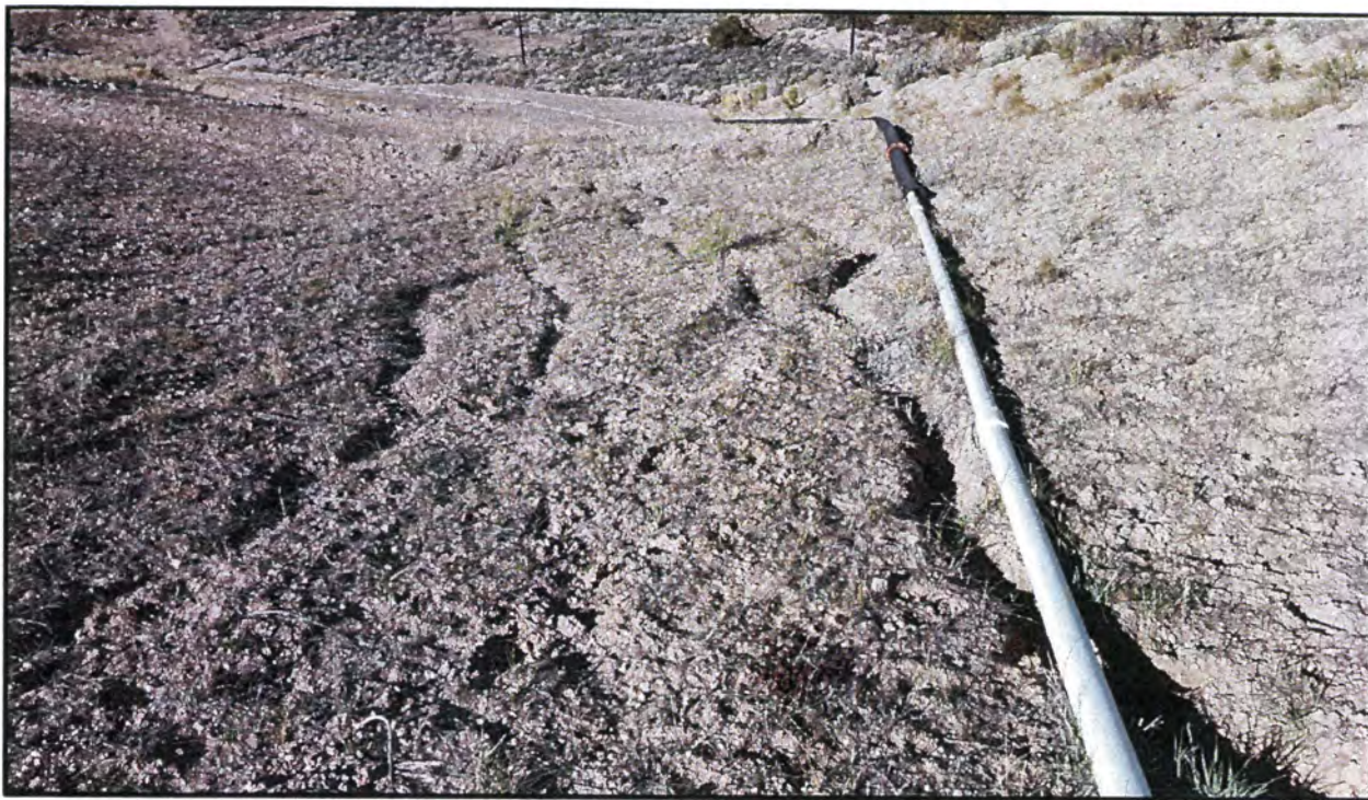
Photo 23 Looking west over minor erosional rilling and gullying developing in recently repaired and re-seeded area at the right downstream groin. (Note white PVC seepage pumpback line at right side of photo.)
