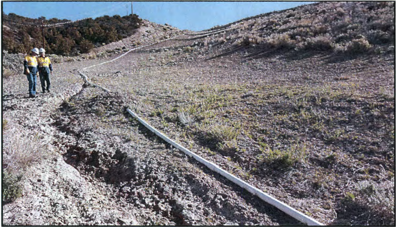
Photo 25 Looking northeast from near the bottom of the right downstream groin. Note erosional gullying and the emergence of new vegetation in the area.
