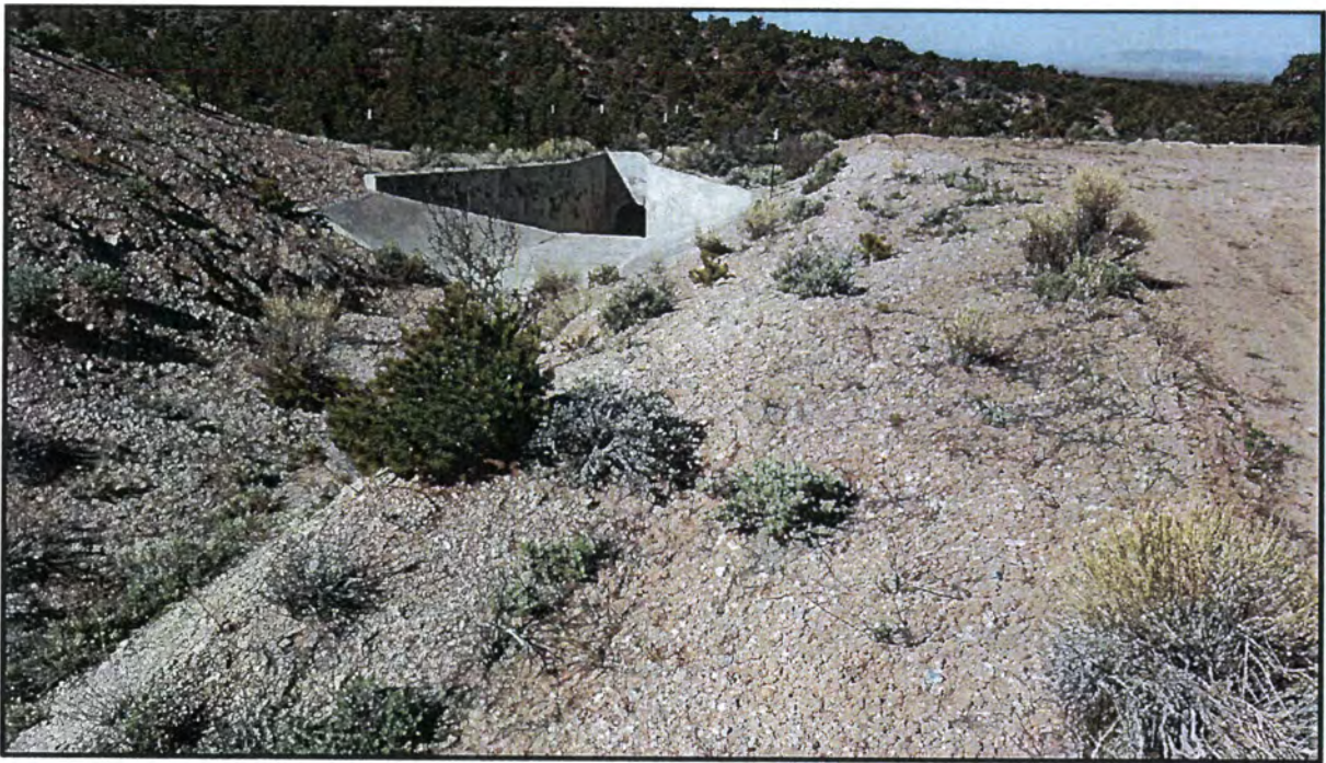
Photo 18 Looking west across entrance to the drop structure for the south diversion channel.
