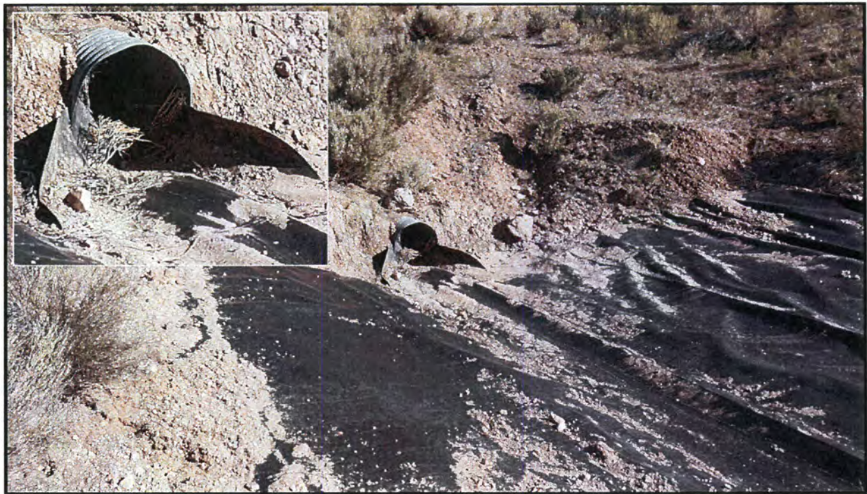
Photo 30 Looking north at the culvert inlet for the access road crossing of the left downstream groin. Note the sediment and brush beginning to accumulate at the inlet.
