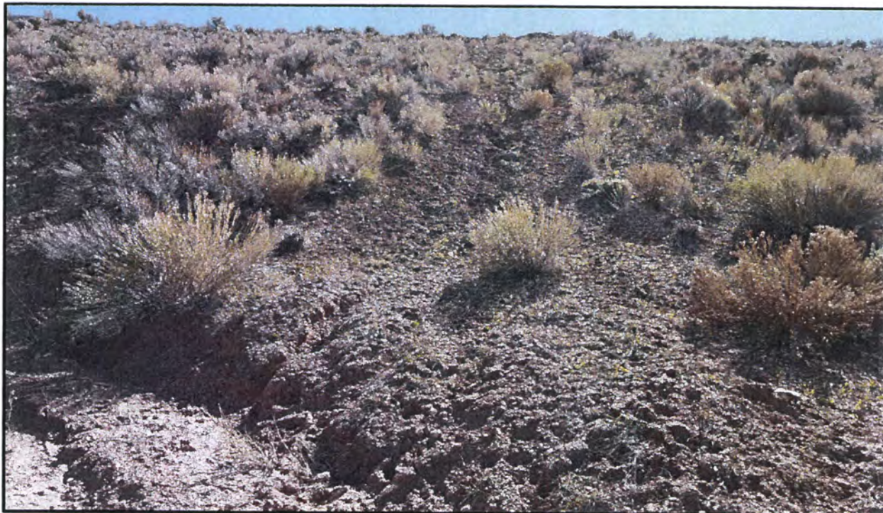
Photo 31 Looking east from the access road just above the left downstream groin, showing development of an erosional gully.
