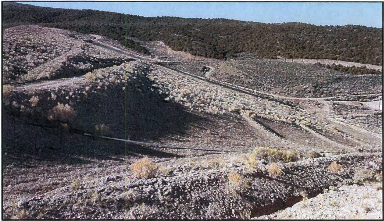
Photo 3 North end of dam, looking southwest over the right downstream groin and downstream face. Note the recently (2016) regraded and re-seeded area in the foreground.
