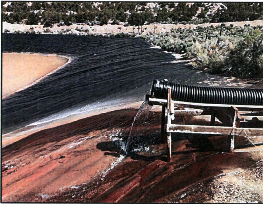
Photo 15 Looking north over toe drain outfall pipe discharging to the seepage collection pond. Note clear seepage discharge.
