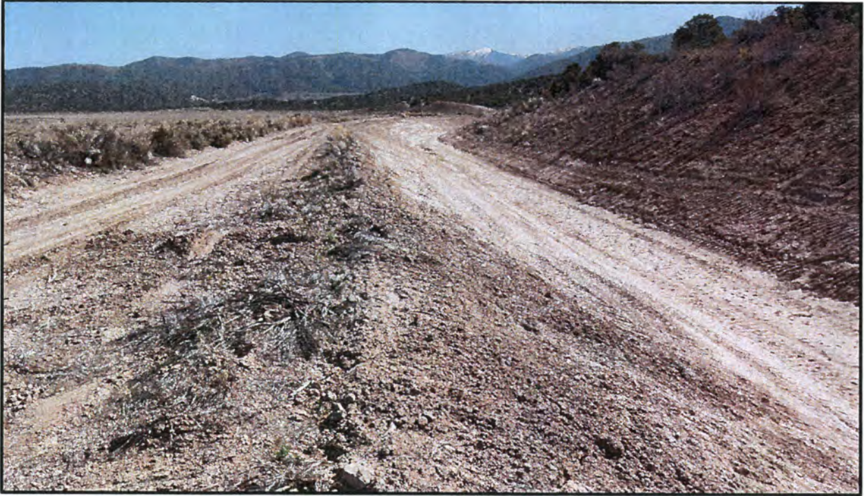
Photo 21 South-central edge of TSF, looking east along the TSF access road and south diversion channel. Note the improved grading in the south diversion channel performed in late 2016 in preparation for 2018 spillway improvements.
