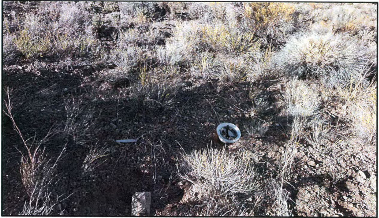
Photo 27 Minor erosional rilling at the lower portion of the downstream face south of the toe drain outlet. Note the hardhat resting in one of the rills.
