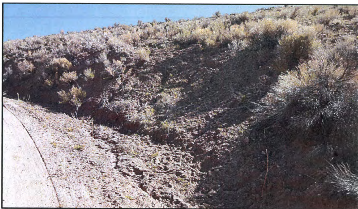
Photo 32 Looking northeast from the access road at the road cut just above the left downstream groin, showing minor erosional rilling.
