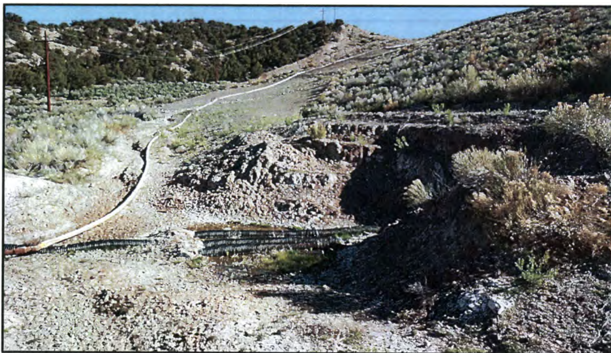
Photo 14 Looking northeast over toe drain discharge pipes, right downstream groin, and right downstream face. Note minor erosional gully near the bottom of the groin along pumpback line.
