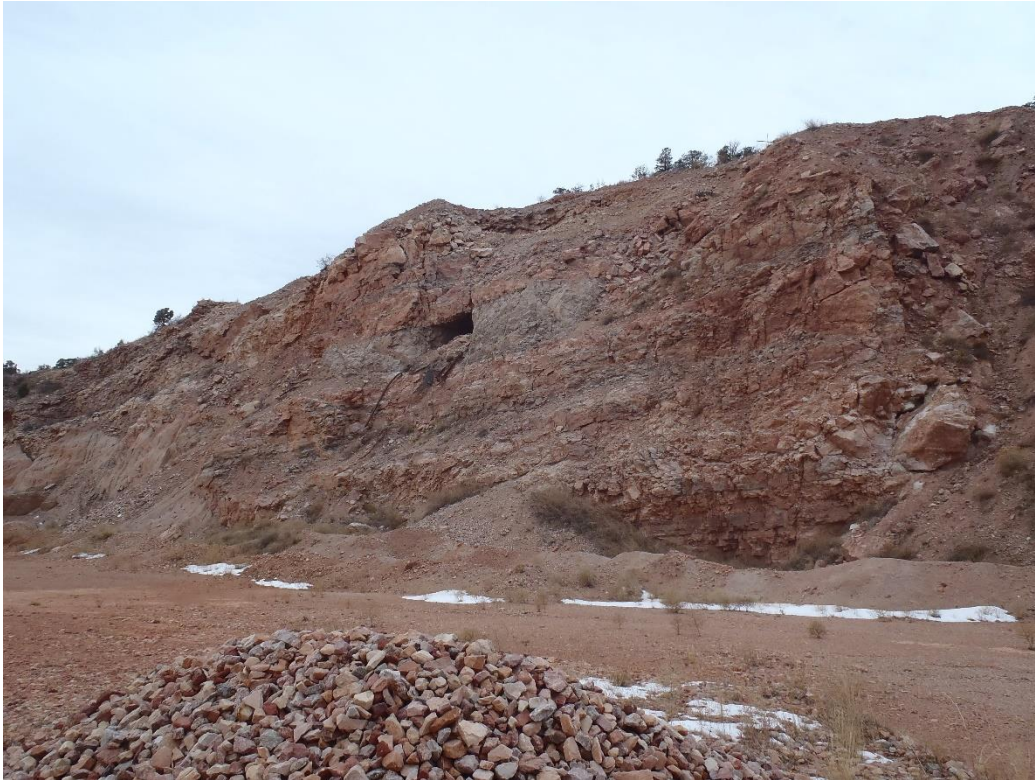
Photo 4. West ridge of WP pit needing benching for final reclamation (looking SW).
