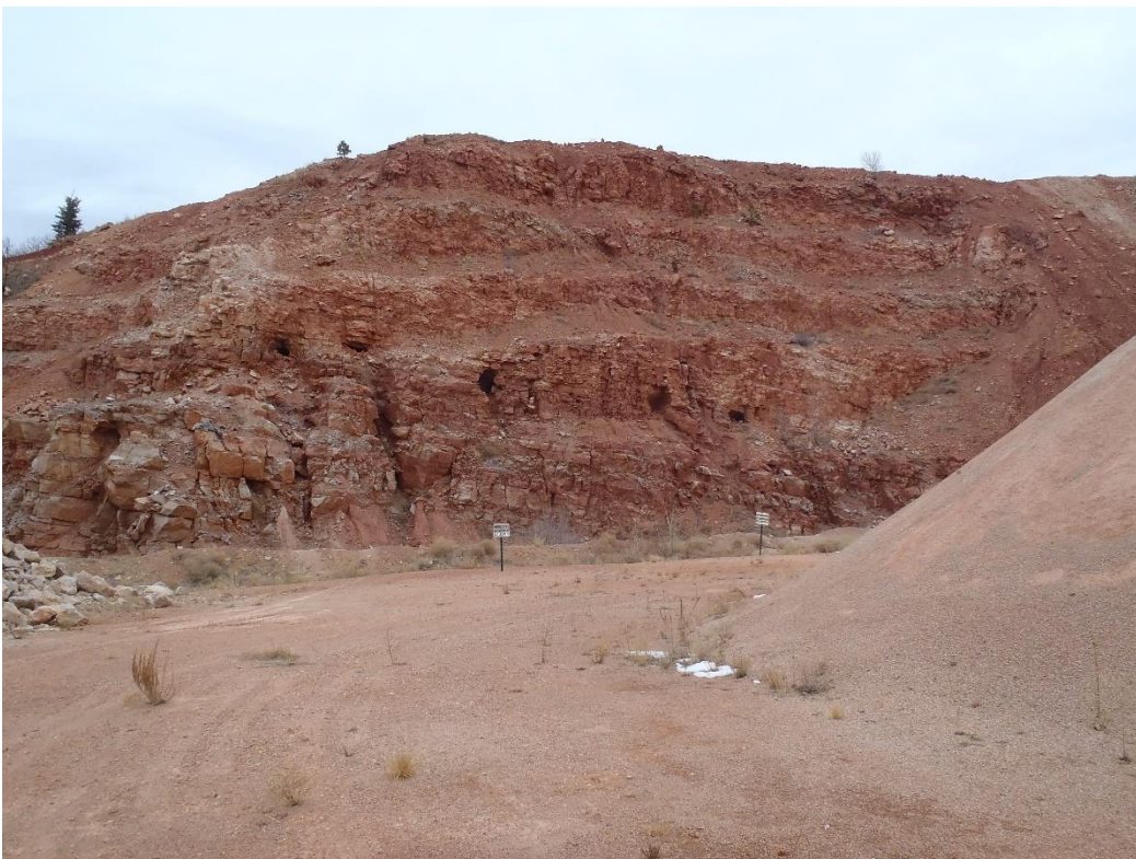
Photo 5. Northeast portion of the WP pit needing benching for final reclamation (looking NE).
