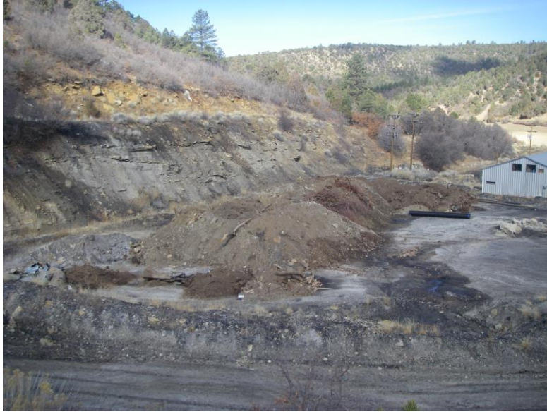
Material from road construction placed on King I facility area
