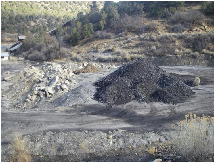
Rock from road construction (on left) and King II mine waste (on right) placed on King I facility area
