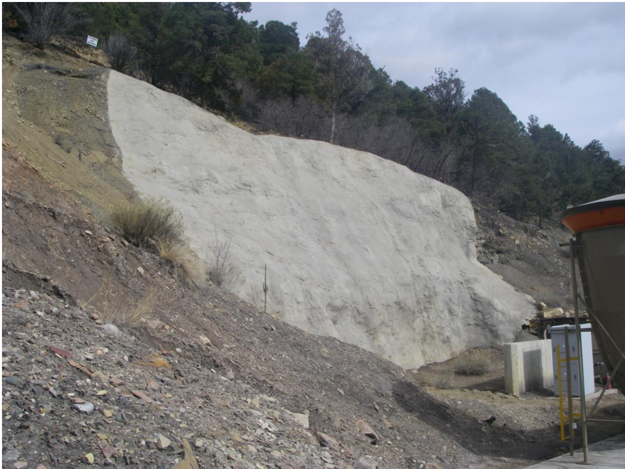
Retaining wall at old fan site
