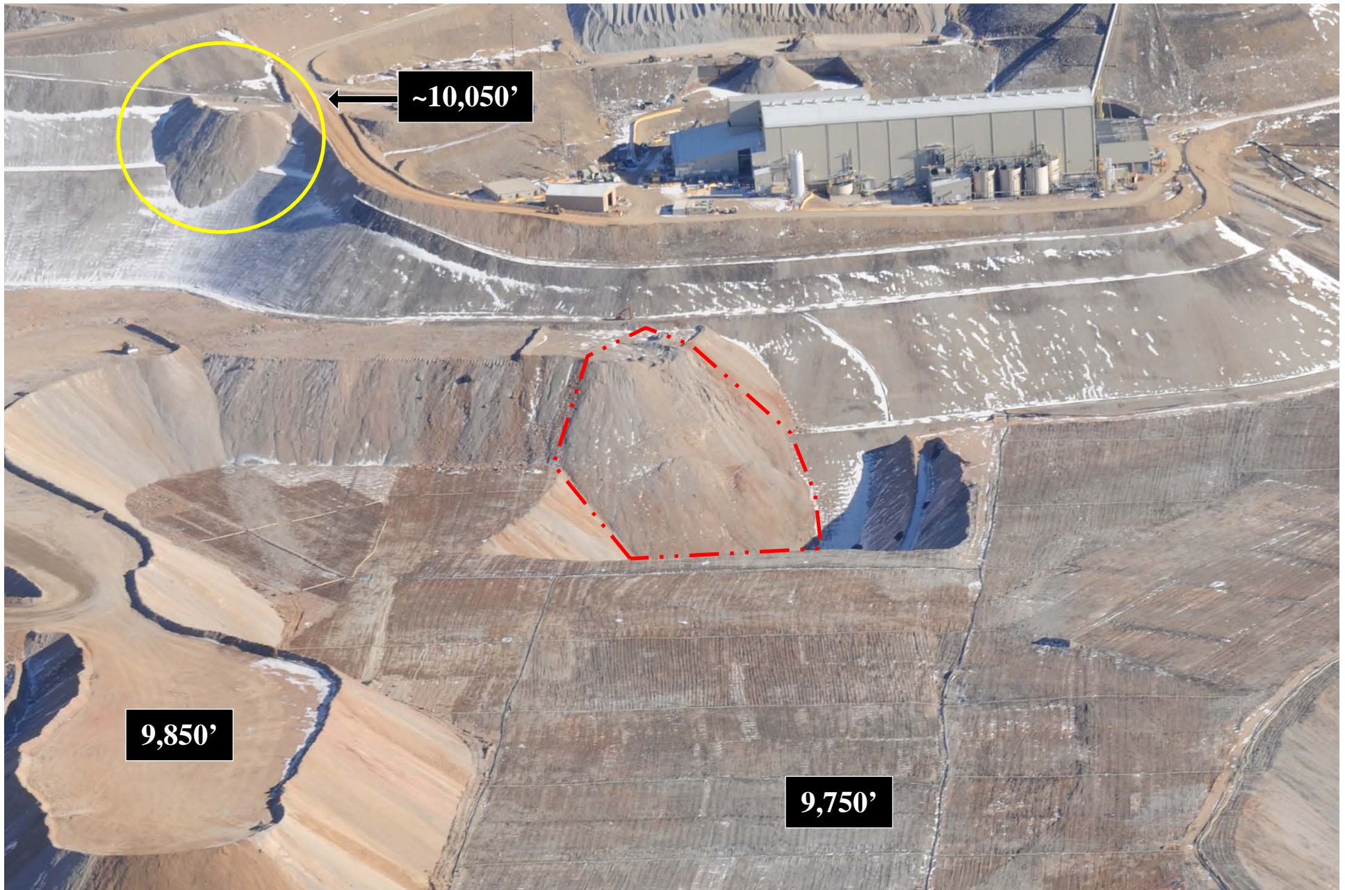
Photo 6. Zoomed in portion of Photo 5, area of slope failure outlined in dash-dot-dot red, approximate 10,050 lift circled in yellow; looking southeast.
