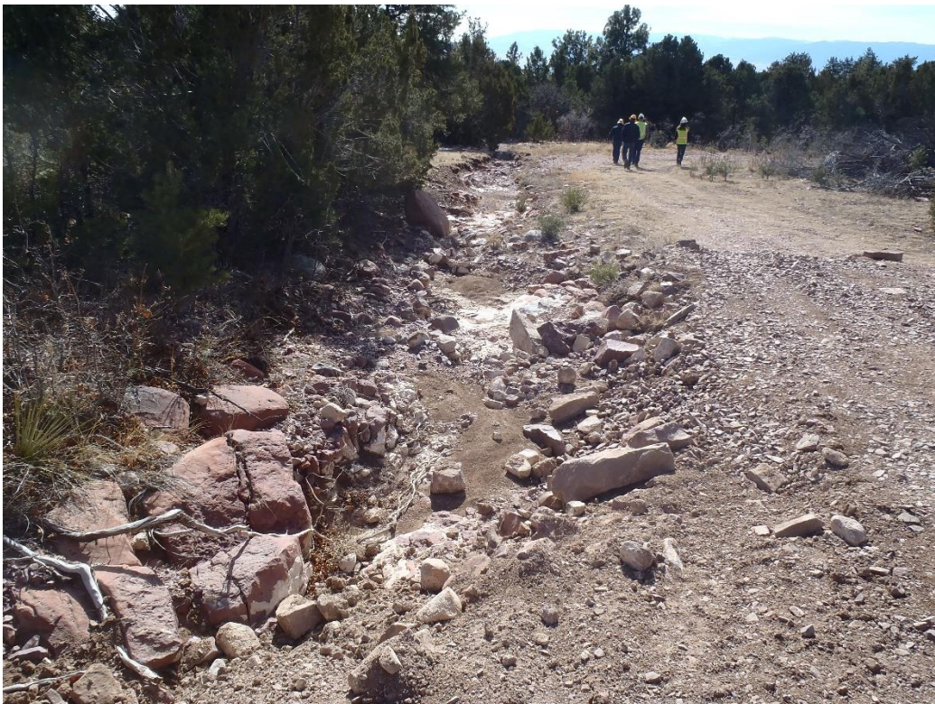
Photo 8. Stormwater channel along road south of sediment pond (looking south).
