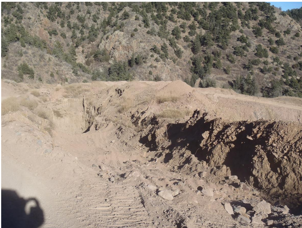
Photo 3. Sediment trap along main haul road (looking NNE).
