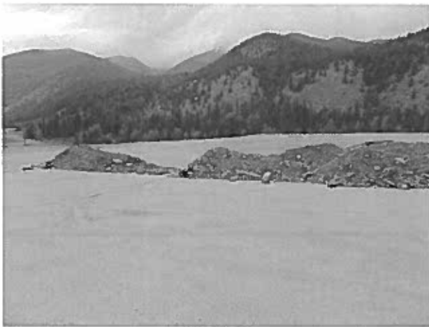
Photo 6. Imported topsoil on graded surface
