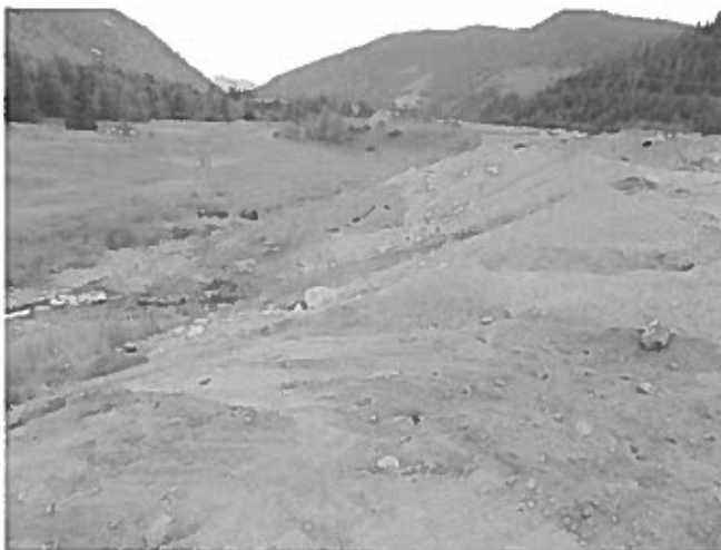
Photo 8. Topsoil spread on the prepared surface.
