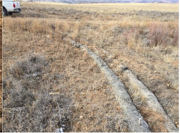
Photo 2 – Erosion Wattles
