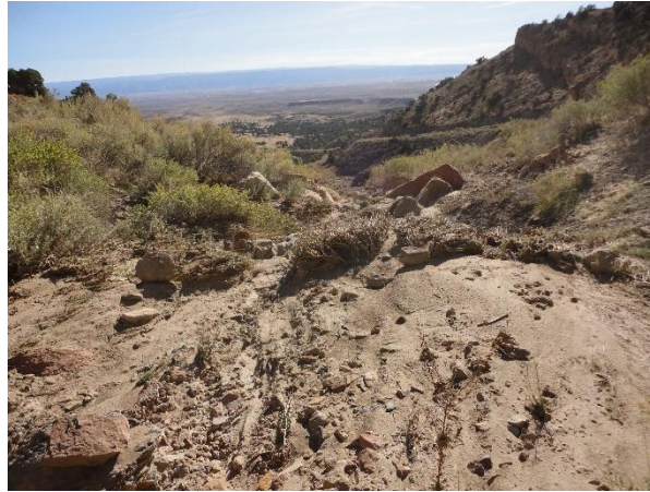
Photo 6: Sediment flow across reclaimed road at Photo 5 Location (looking SE)
