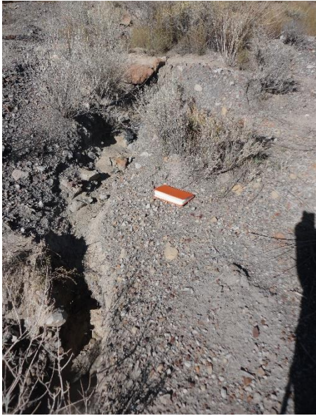
Photo 1: rill formation at base (south end) of road
