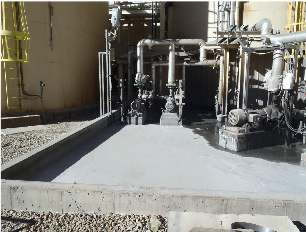
Photo 2. Neutral Process Water Tank secondary containment area.
