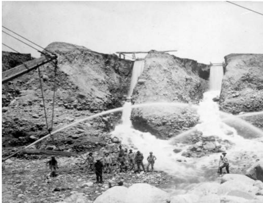
Hydraulic mining the Alma Placer, Alma, CO
