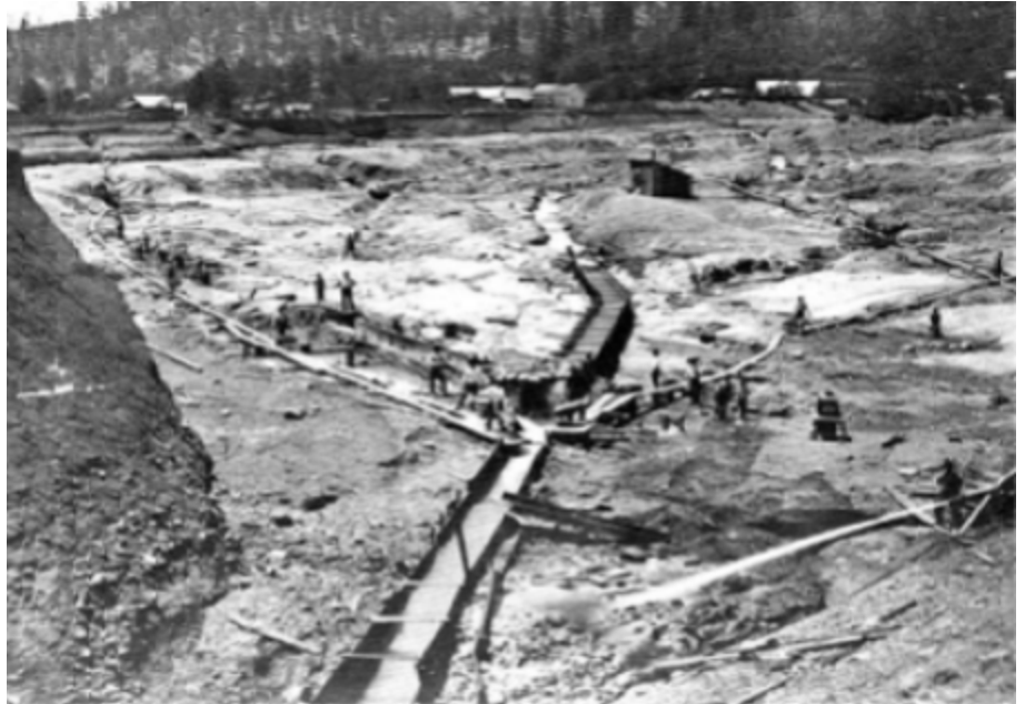
Above: Elaborate sluice and trough system
