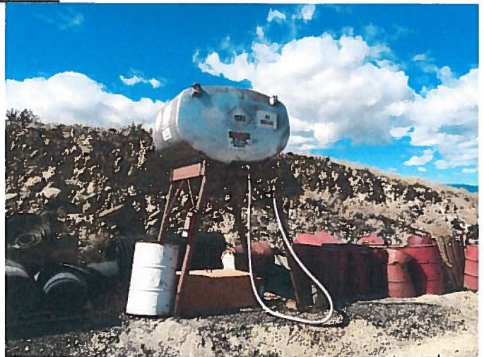
Fuel Storage with no secondary containment- PROBLEM
