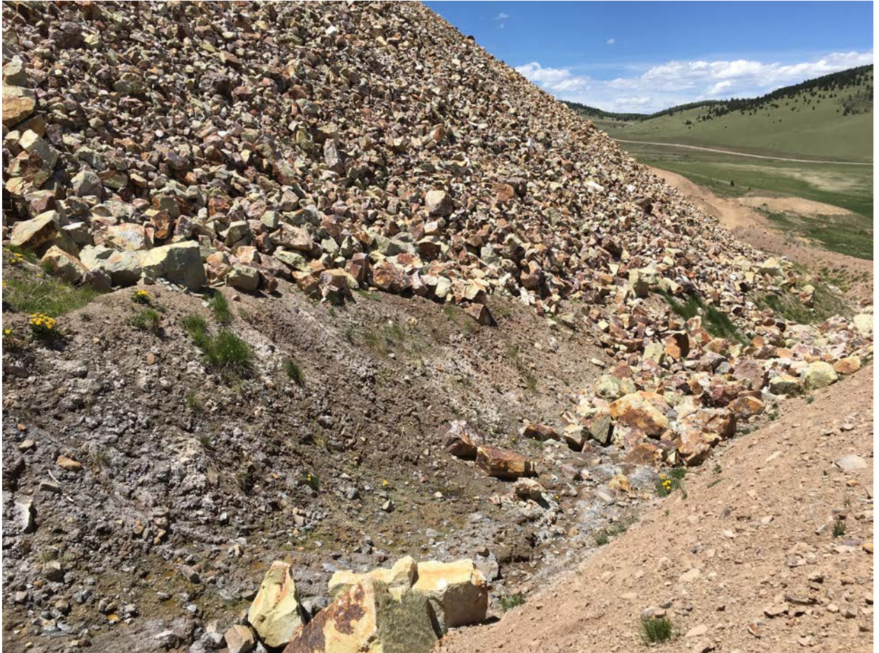
Photo 1. Seep identified at toe of ECOSA 15 June 2017. Photo looking northeast at south-southeast side of the ECOSA.
