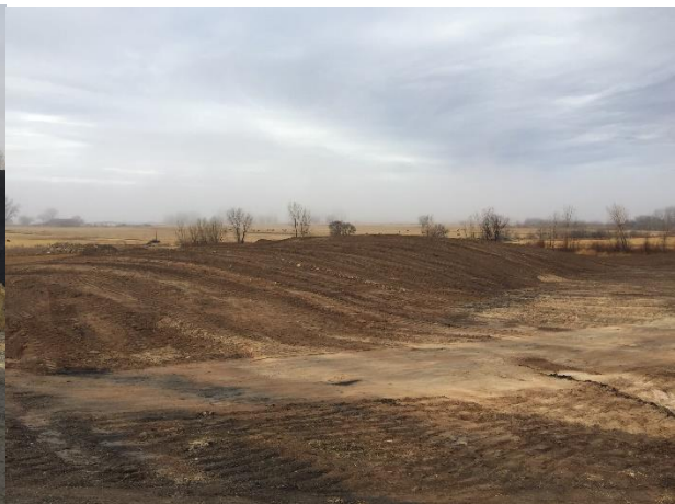
Photo 4 – Topsoil Salvaged Ahead of Coal Pile
