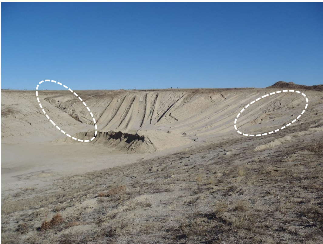
Photo 1. Rills and gullies in the active face (looking NE).
