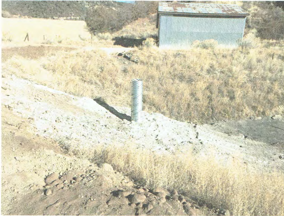
Pic. 3 – New outlet structure East Pond.
