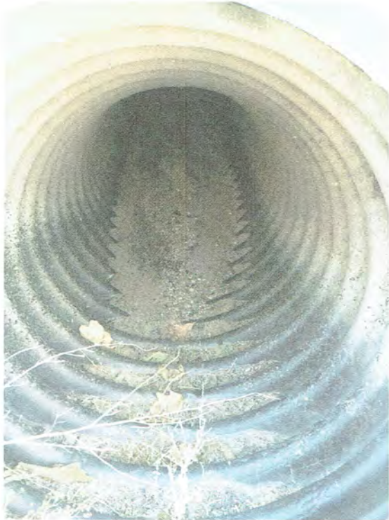
Pic. 5 – Some sedimentation in base of corrugated plastic pipe.
