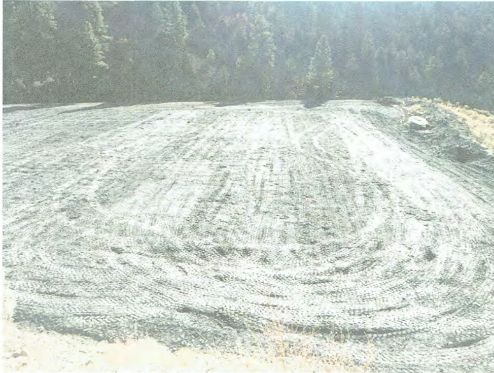
Pic. 5 – Embankment material has been placed at the top of the waste pile.
