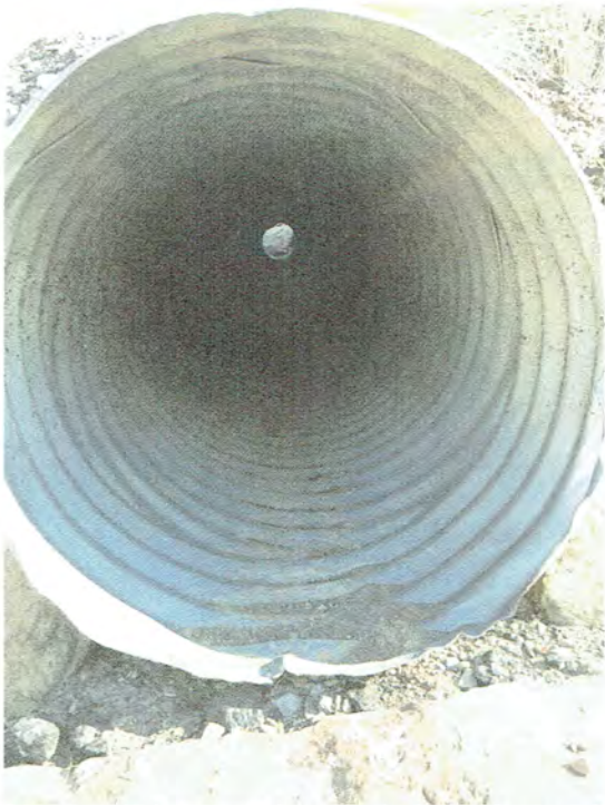
Pic. 2 – Culvert under road above base of embankment.
