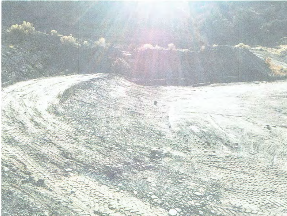
Pic. 3 – Additional material installed at base of embankment/waste pile.
