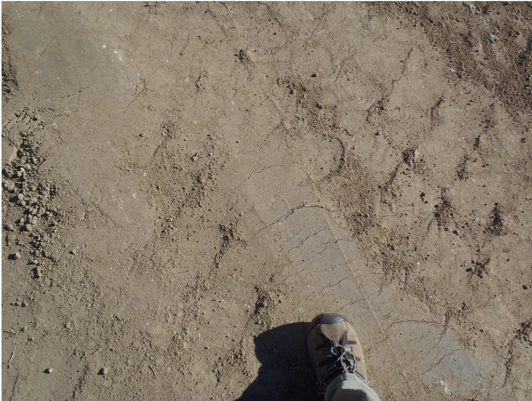
Photo 6. Heavily compacted soil in second from west gully repair.
