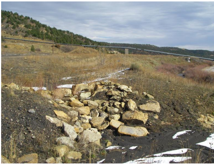
Riprap below SAE near Topsoil Stockpile #2 (note sediment in lower right portion of photograph)
