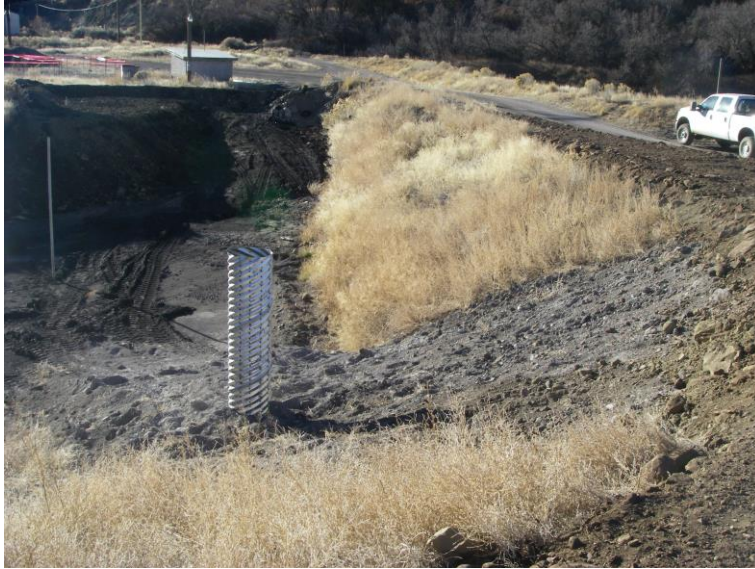
East Pond (King I) – new primary spillway
