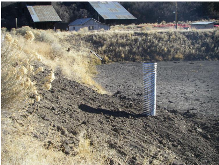
King I West Pond – new primary spillway
