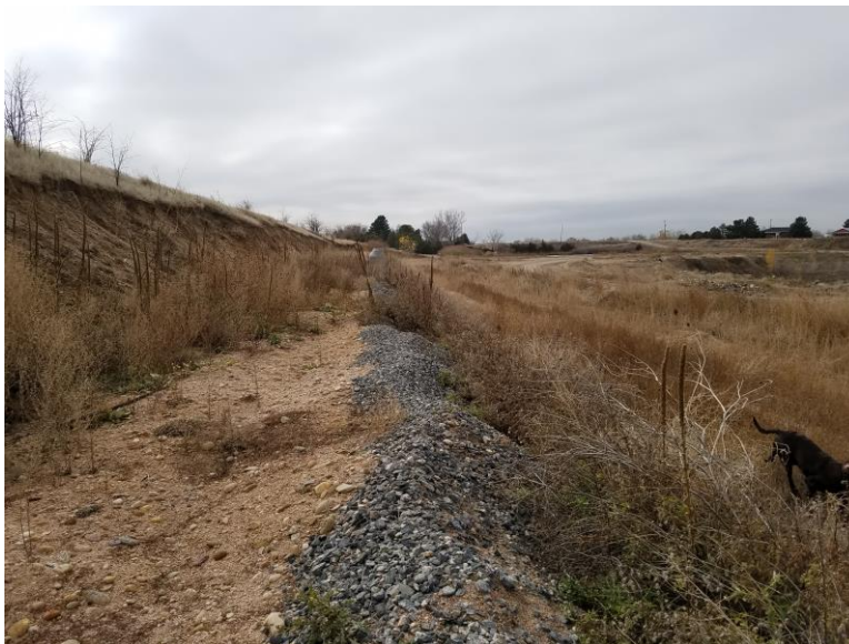
Figure 14. French drain installed on the east side of Pit 2.
