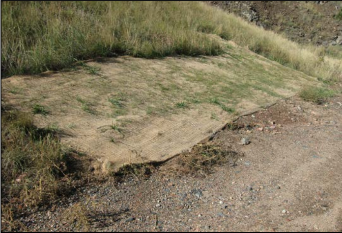
1. Erosion repair to South Waste Rock Pile.
