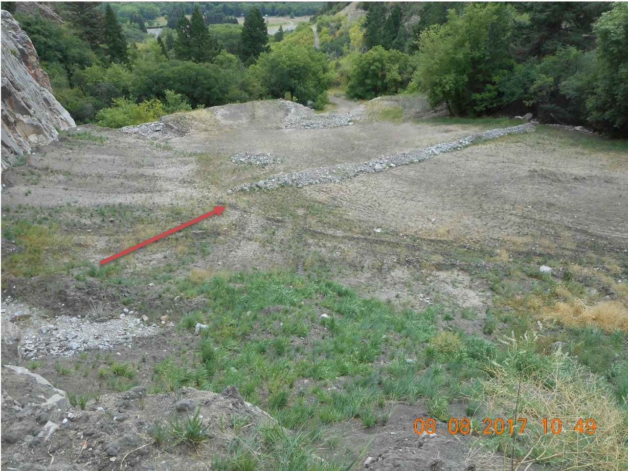
Photo 4: Looking southeast from the reclaimed upper quarry bench. Note the slight gully beginning to form around the northern (left) side of one of the windrows (red arrow).
