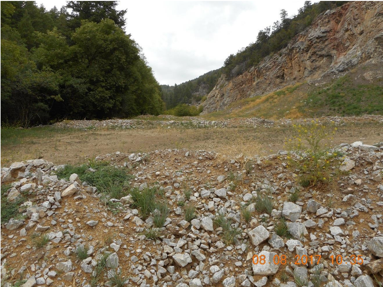
Photo 3: Looking west at the sediment control windrows that run north-south (right to left) across the quarry floor. The unknown mustard plant species is located in the right foreground.
