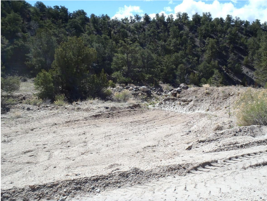
Photo 10. Another sediment trap (along haul road).
