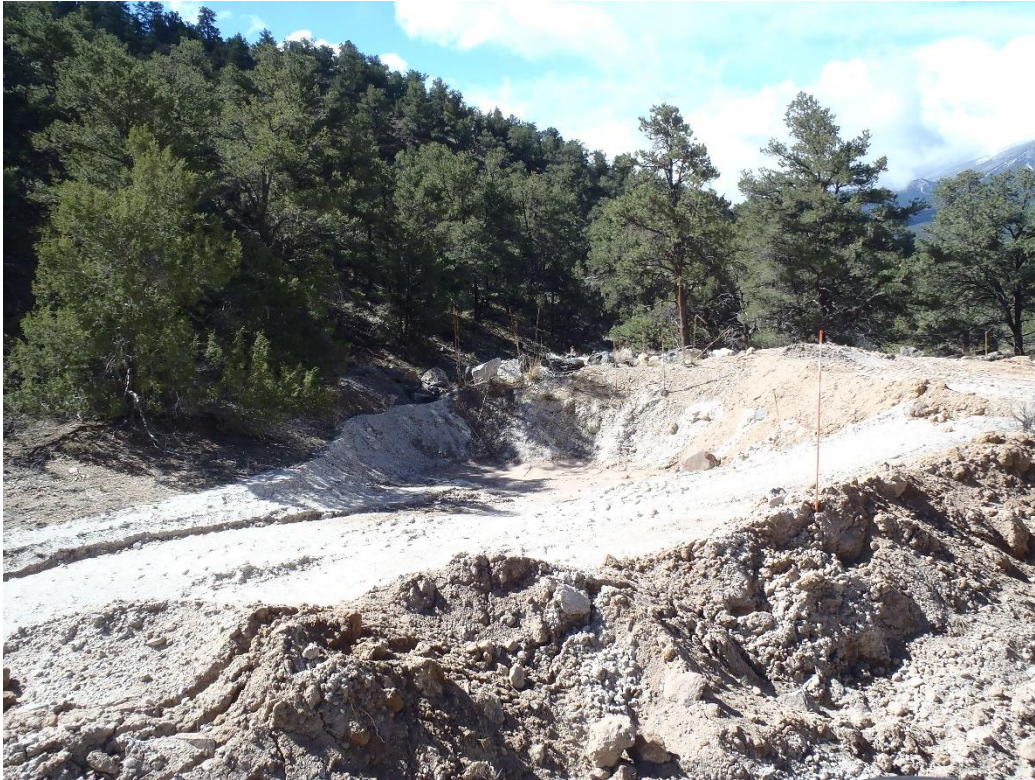
Photo 4. Typical sediment trap (along haul road).
