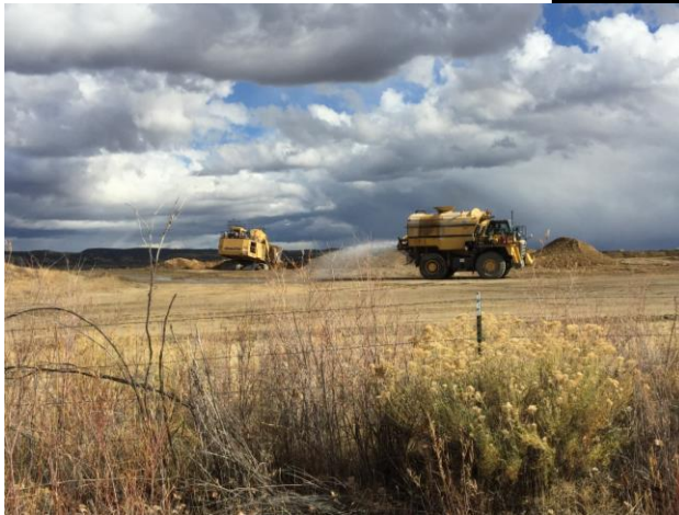
Photo 1 – Watering Pit Roads for Dust Control
