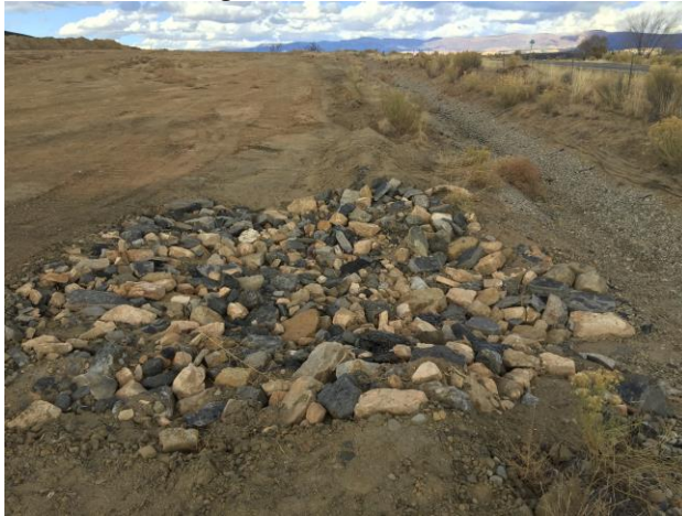
Photo 3 – Rock Lined Spillway
