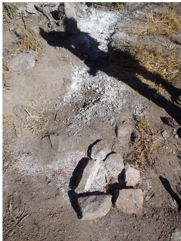
Photo 5. Grout overflow was observed at WG-16-36.
