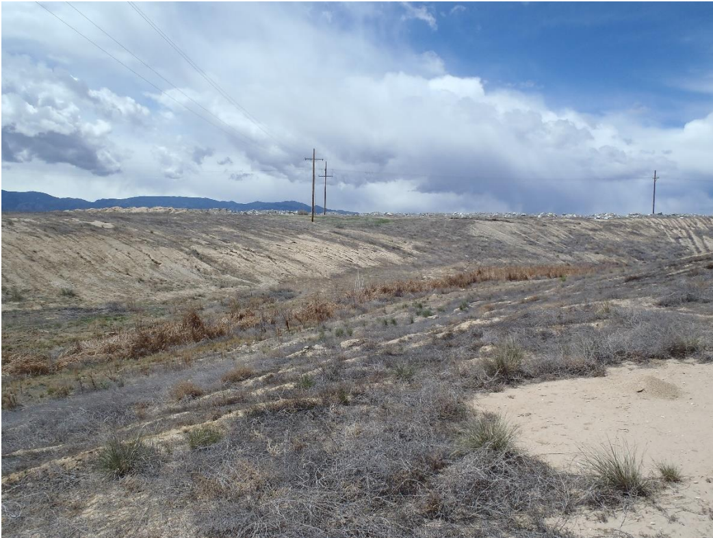
Photo 7. Erosion rilling / gullying observed along Bear Creek realignment (looking NW).
