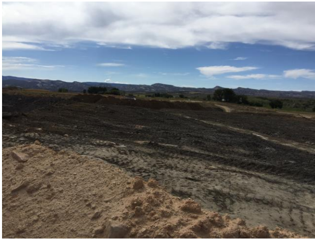
Photo 1 – Backfill in Center of Pit
