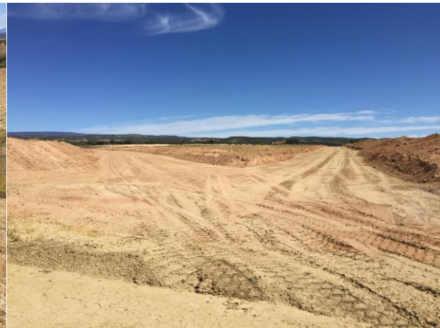
Photo 4 – Topsoil Moved for CCC Ditch Install
