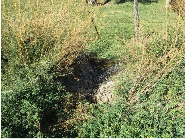
Photo 1 – Gabion Cage Sediment Control
