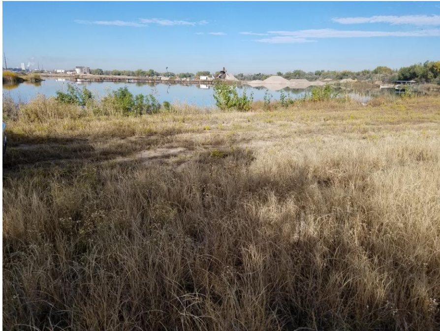
Figure 3. Approximate location of where the eastern pit slope breached.
