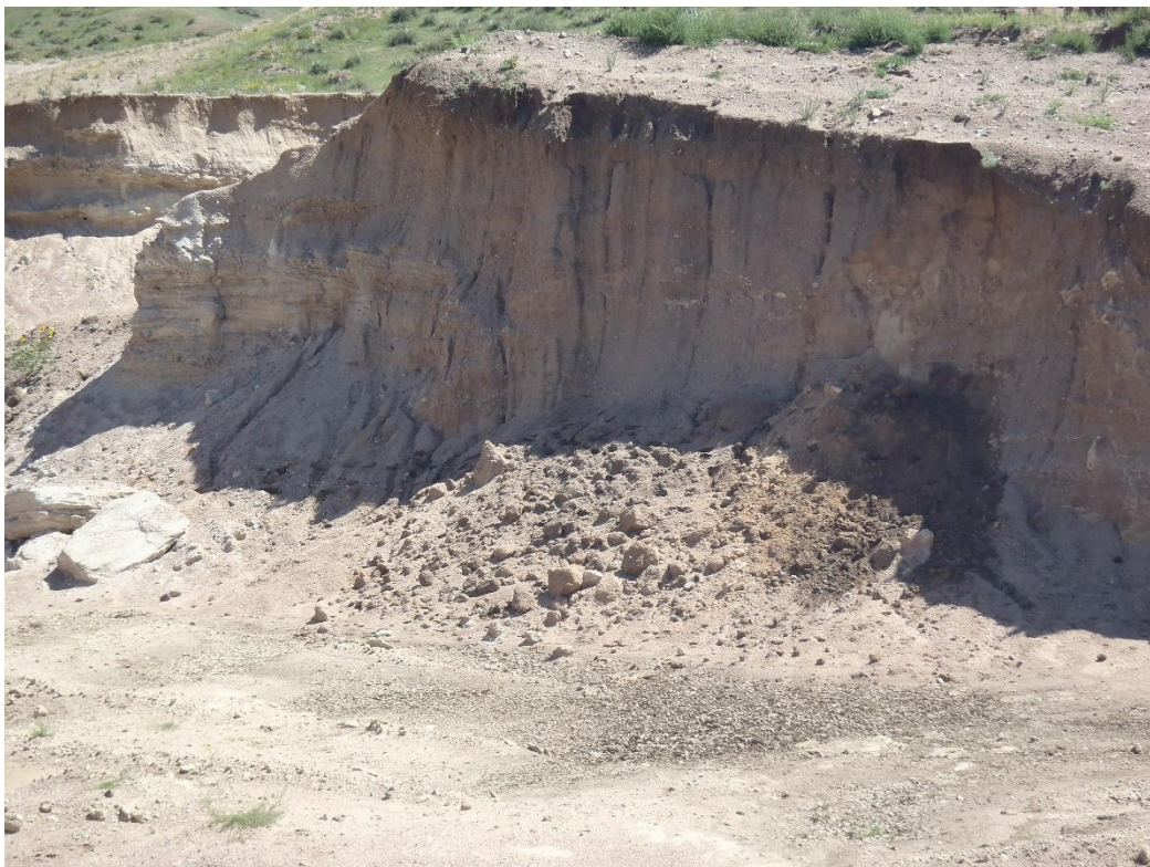
Photo 3. Less stable internal highwalls (with respect erosion), but not considered problematic.
