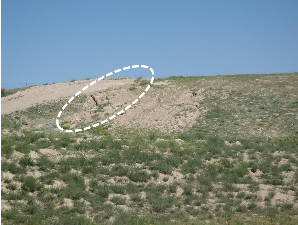
Photo 4. Large erosion gully observed along the haul road (looking NW).
