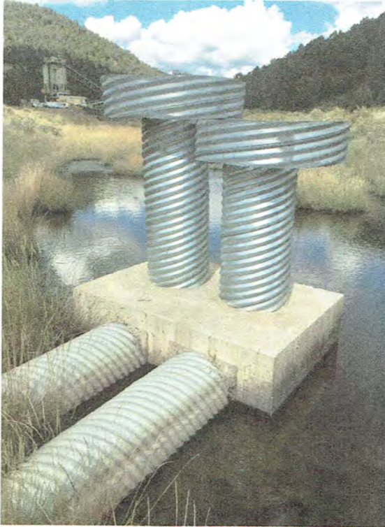
Pic. 1 – Detention Pond with 2-inches of water at outlet structure.
