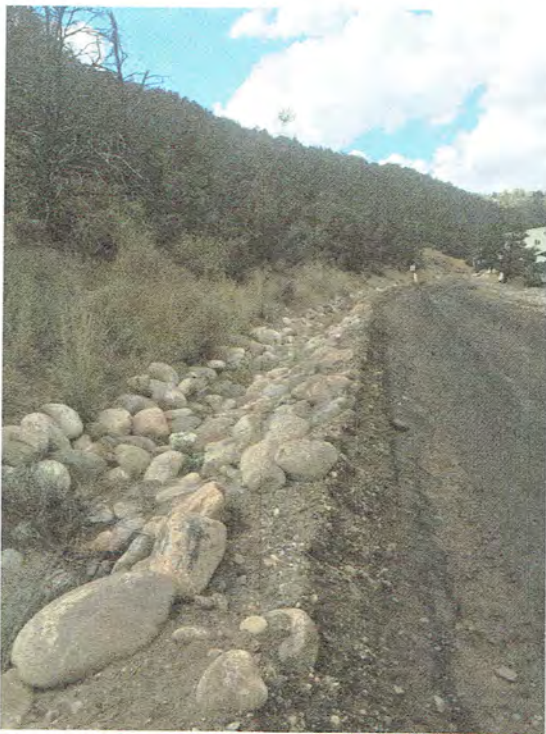
Pic. 4 –West clean water ditch has been cleaned.
