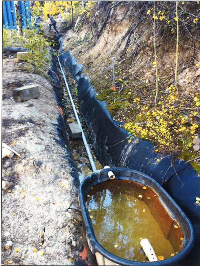
Photo 5. View looking upslope from the post-filtration sediment basin towards the slag filter. Outlet from sediment to basin to Deadman's Gulch and the lower sump is shown at the bottom of the photo.
