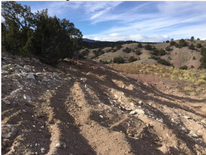
Photo 5: Showing the loose material used to backfill the highwall.
