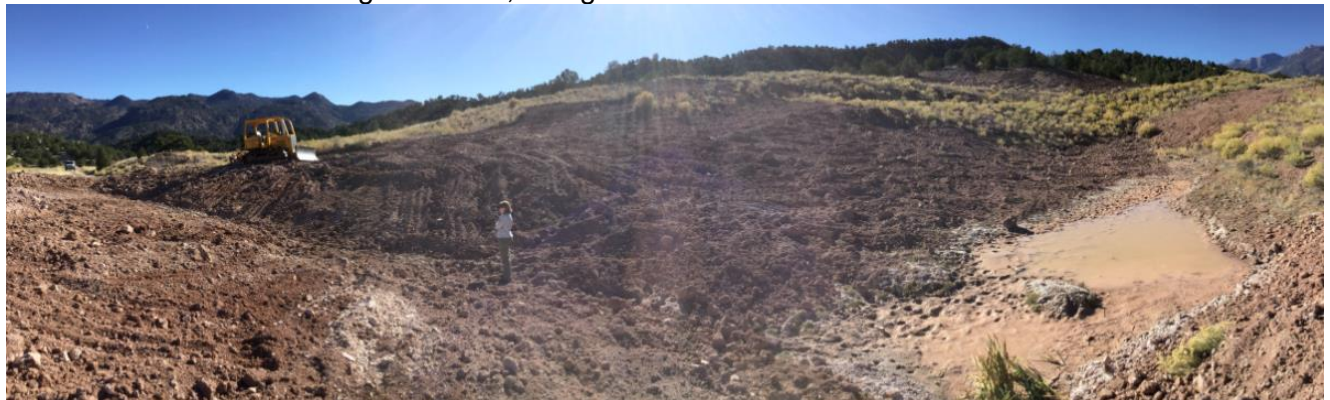
Photo 1: Panorama showing the swale, and grader.
