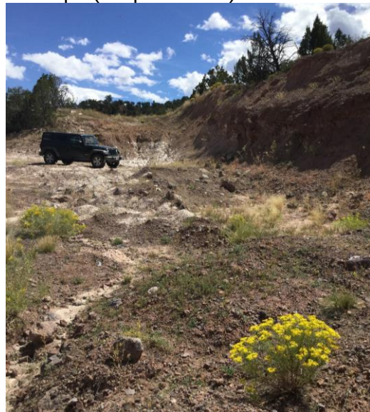
Photo 2: The clay mine highwall to be reclaimed to a 3:1 slope (Jeep for scale).
