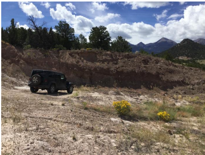
Photo 2: The clay mine highwall to be reclaimed to a 3:1 slope (Jeep for scale).
