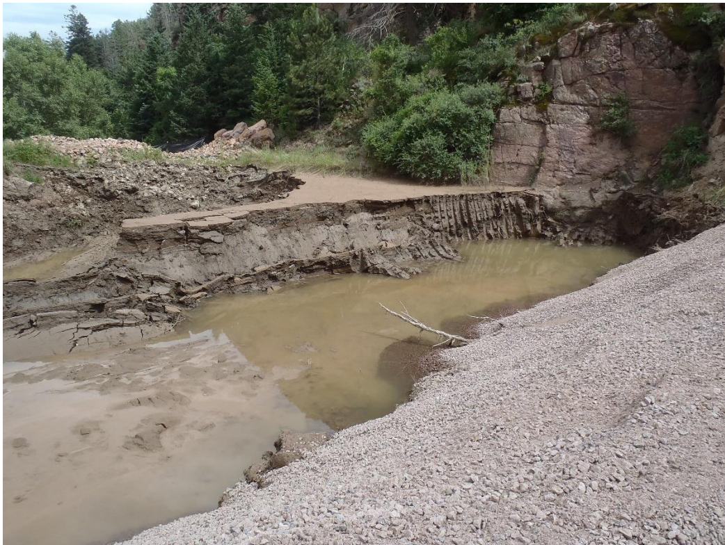
Photo 3. Sediment pond in the process of being mucked out.
