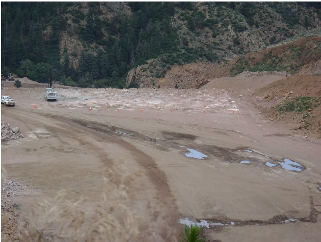
Photo 1. Drilled blast pattern (looking east).
