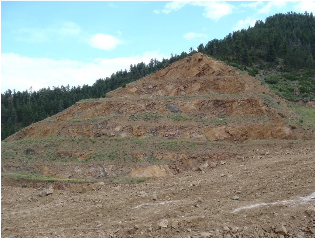
Photo 2. South side highwall benches in reclamation.
