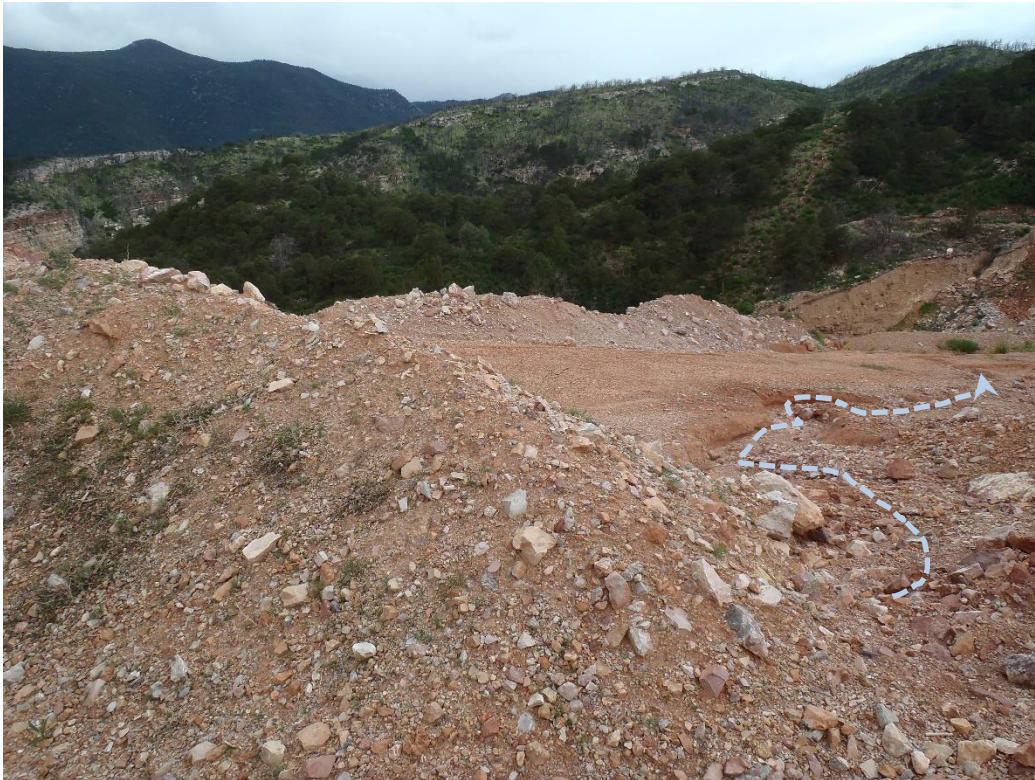
Photo 5. Erosion gully in haul road between north and south pits.
