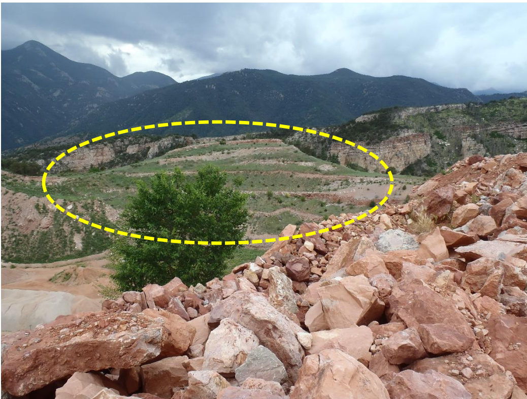
Photo 4. Reclaimed benched west highwall – south pit (looking west).
