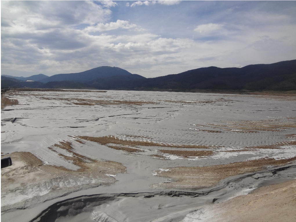
View of deposition cell between leadoffs 5 and 6 on 1-Dam looking southwest
