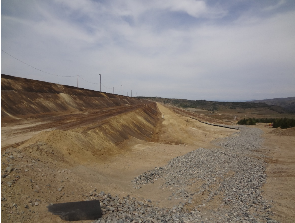
View of rock lined channel in the south groin of 1-Dam looking north
