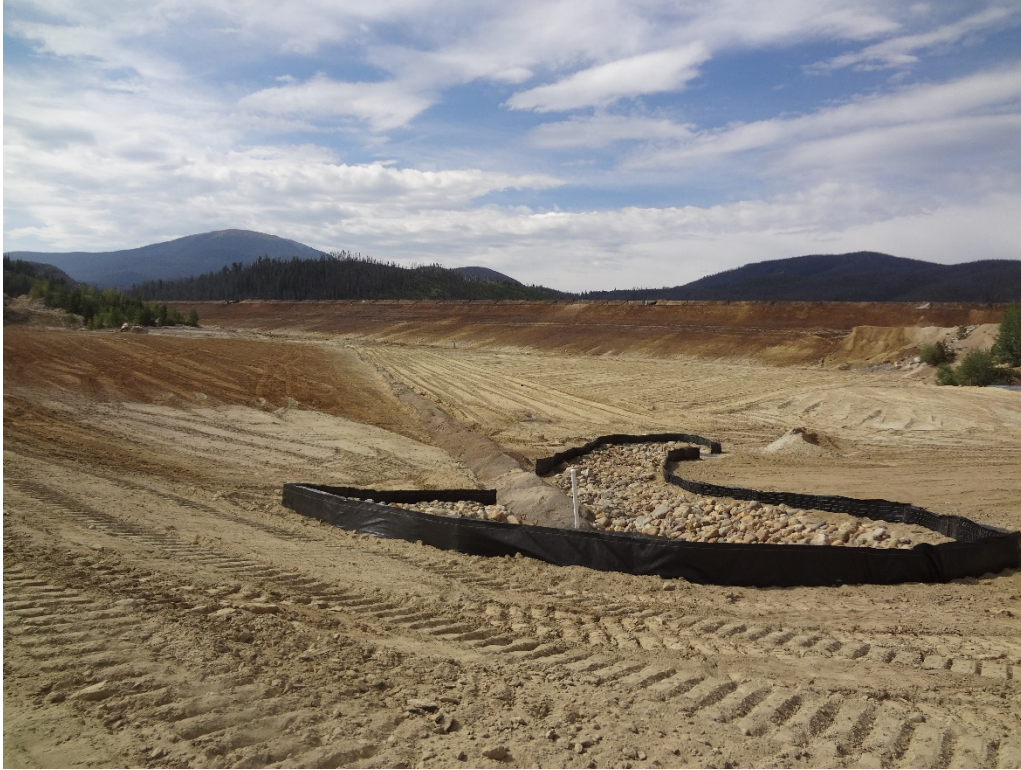
View of north setback bench on the 3 Dam embankment
