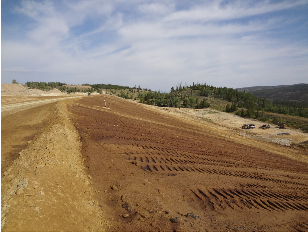
View of the completed 3-Dam embankment regrading work looking north with horizontal drain installation at toe
