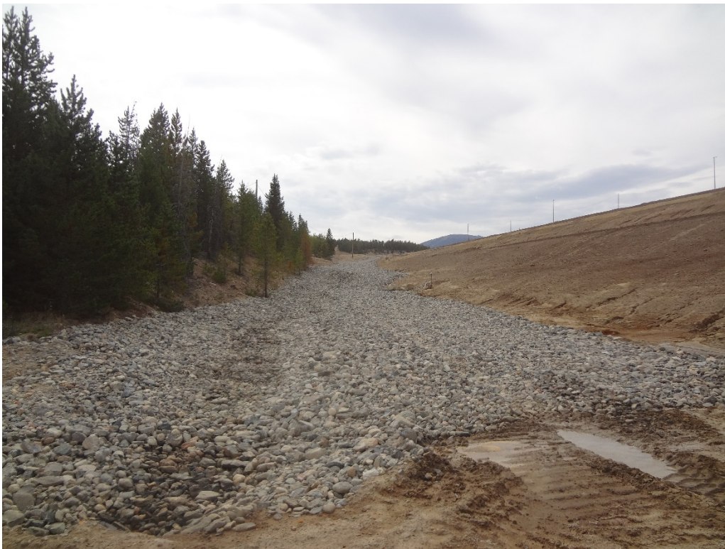
View of rock lined channel in the south groin of 1-Dam looking southwest
