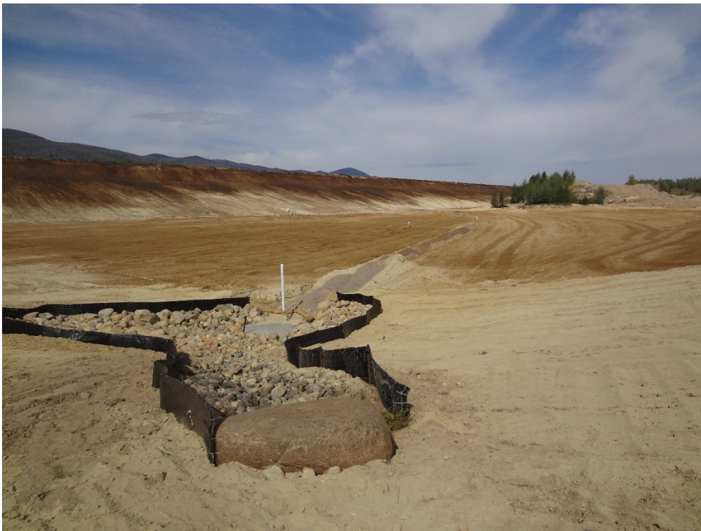
View of south setback bench on the 3 Dam embankment
