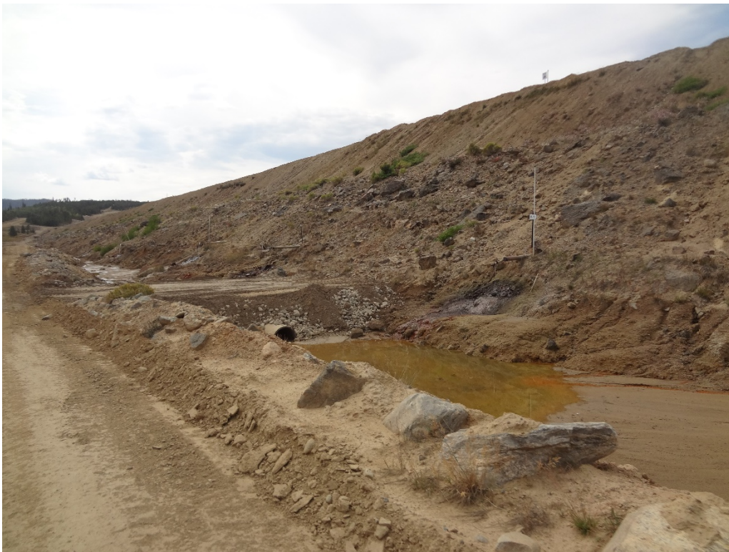
View of horizontal drain drilling pad in 1-Dam
