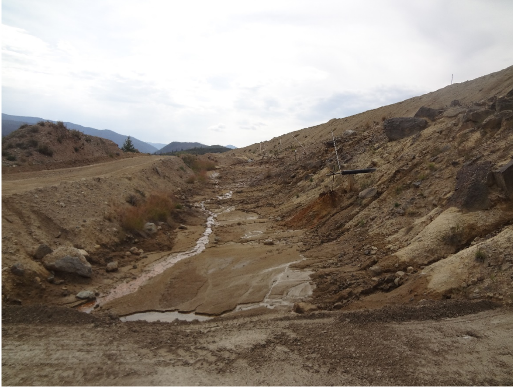
View of seepage collection ditch below 1-Dam looking south
