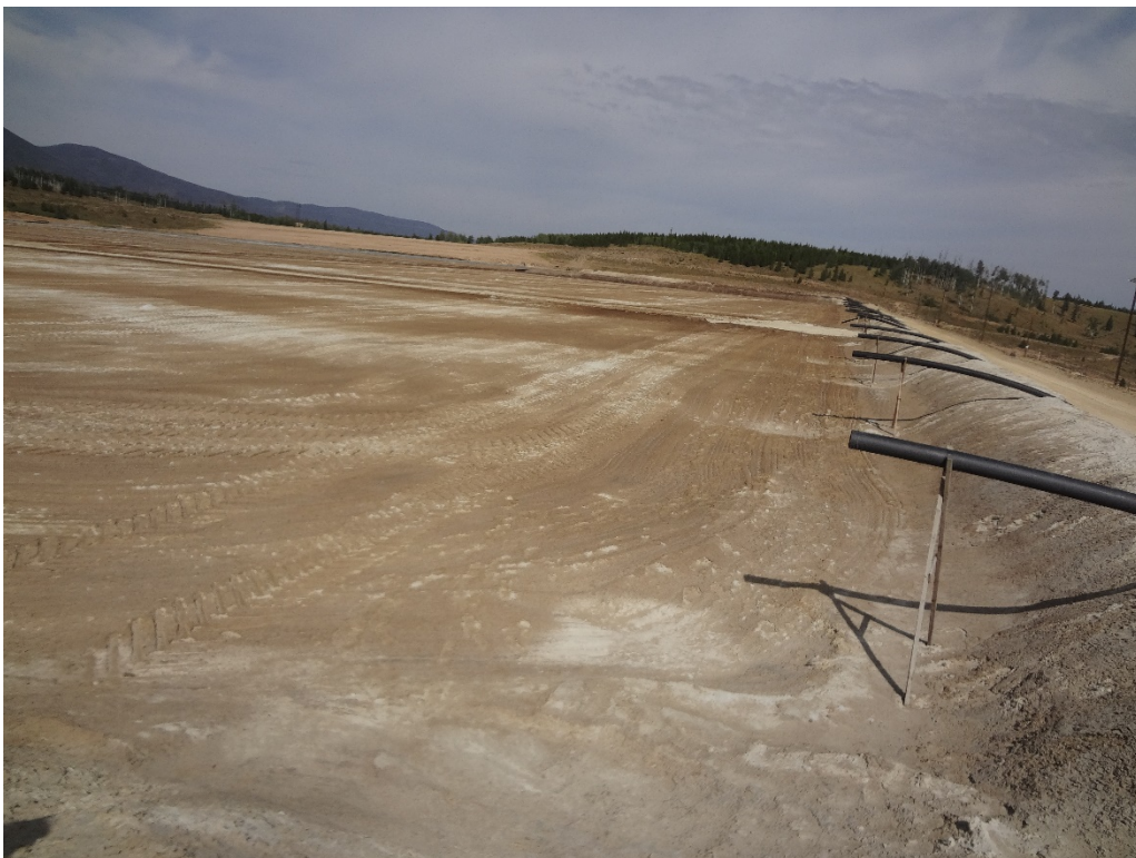
View of deposition cell between leadoffs 6 and 7 on 1-Dam looking north
