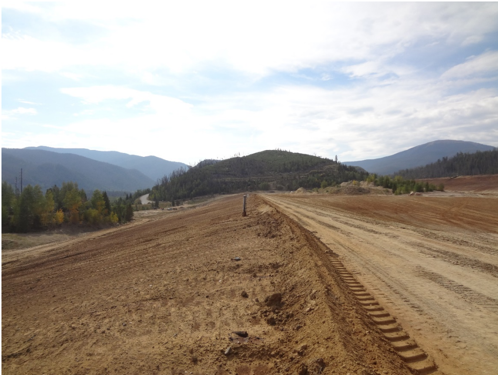
View of the completed 3-Dam embankment regrading work looking south
