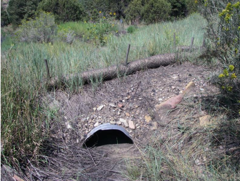
King II – culvert in topsoil stockpile ring ditch
