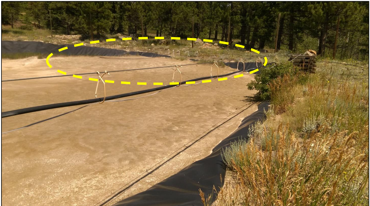
Photo 25. View looking across eastern portion of lined tailings impoundment. Note available freeboard along eastern edge is less than the required two feet (particular area of concern circled).
