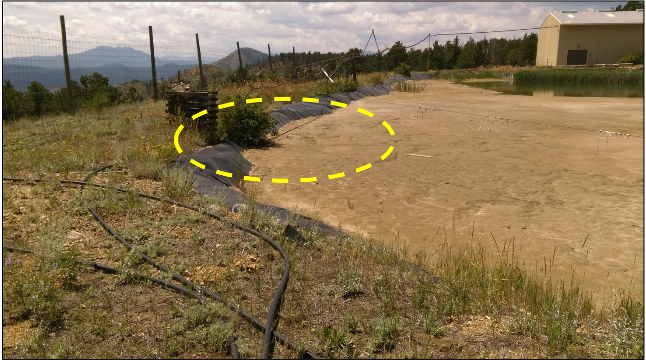
Photo 28. View looking across southern edge of lined tailings impoundment showing portions where available freeboard is less than the required two feet (particular area of concern circled).
