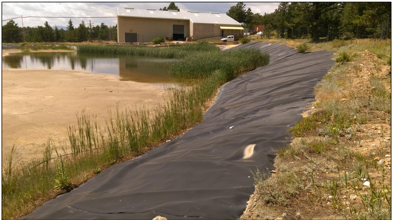
Photo 29. View looking across northern edge of lined tailings impoundment showing available freeboard exceeds the required two feet.
