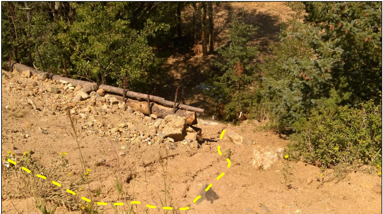
Photo 4. View looking down from northern edge of Sunshine Canyon Drive at Times Mine subsidence area. Approximate edge of subsidence feature (not visible due to fill placement) is indicated with a yellow dashed line. Note fill being held in place by temporary retaining wall composed of timbers stacked between stakes.
