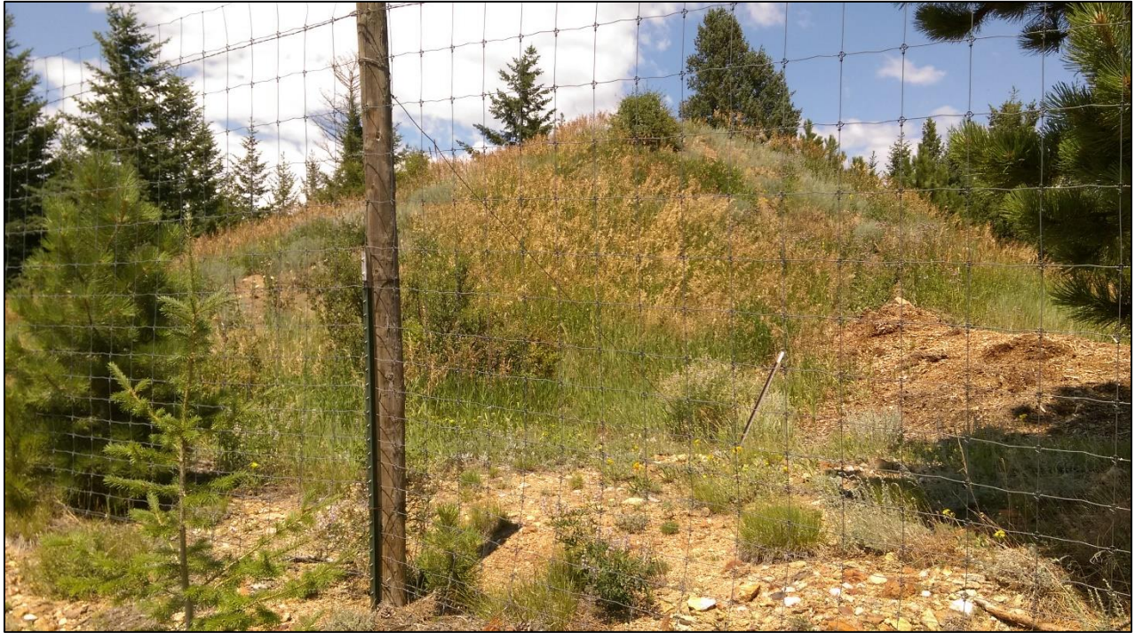
Photo 30. View of topsoil stockpile stored north of tailings impoundment, outside of fenced enclosure. Note stockpile is well vegetated and stable.
