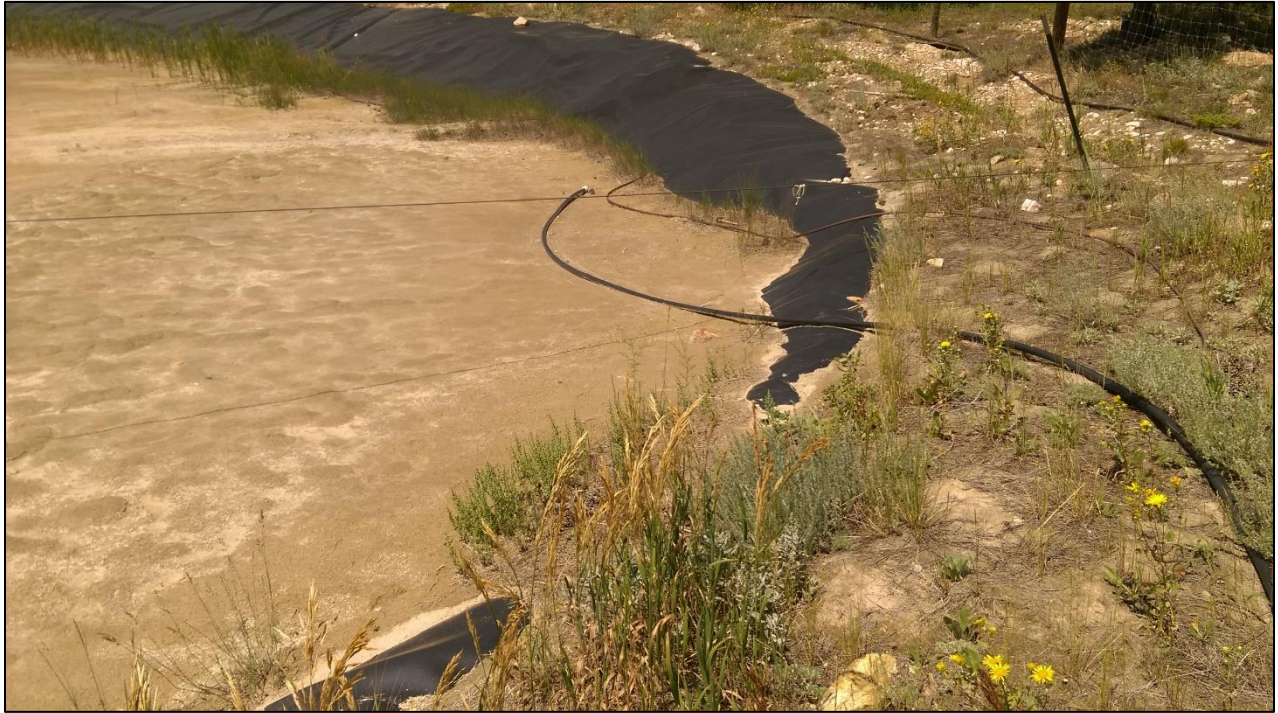
Photo 26. Closer view of eastern edge of lined tailings impoundment showing available freeboard is less than the required two feet.
