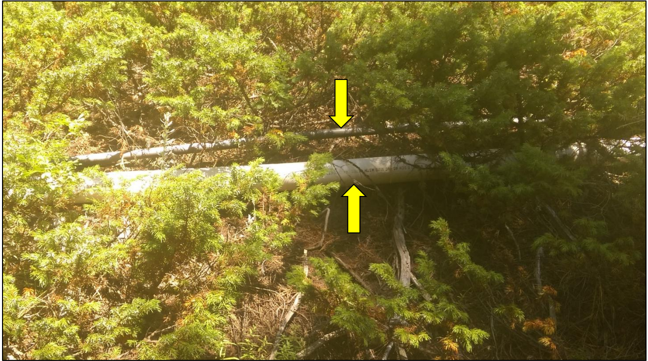
Photo 9. Closer view of two existing pipelines (indicated with arrows) present along edge of trail in Lick Skillet Gulch. According to Mr. Steen, PVC pipe was installed by him when mill was first constructed in 1980's, and smaller black HDPE pipe was installed by previous operator in 1990's.
