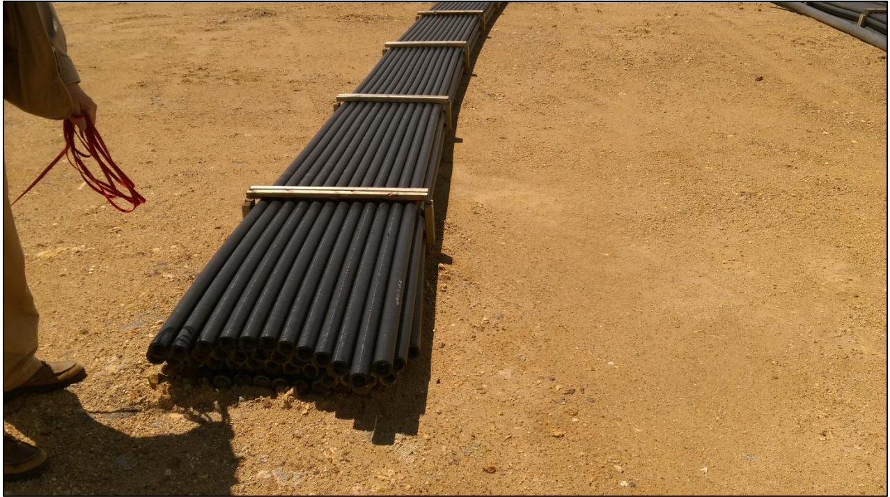
Photo 11. View of one of two stacks of black two inch HDPE pipe currently stored on top of ore stockpile in mill permit area. This pipe is intended to replace two existing pipelines present in Lick Skillet Gulch in order to convey water pumped from Left Hand Creek to the mill.
