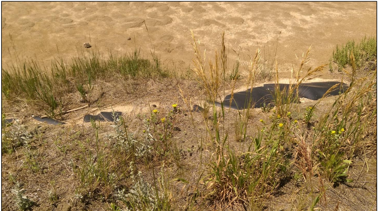
Photo 27. Close-up of portion of eastern edge of lined tailings impoundment where tailings are at or near top of liner.
