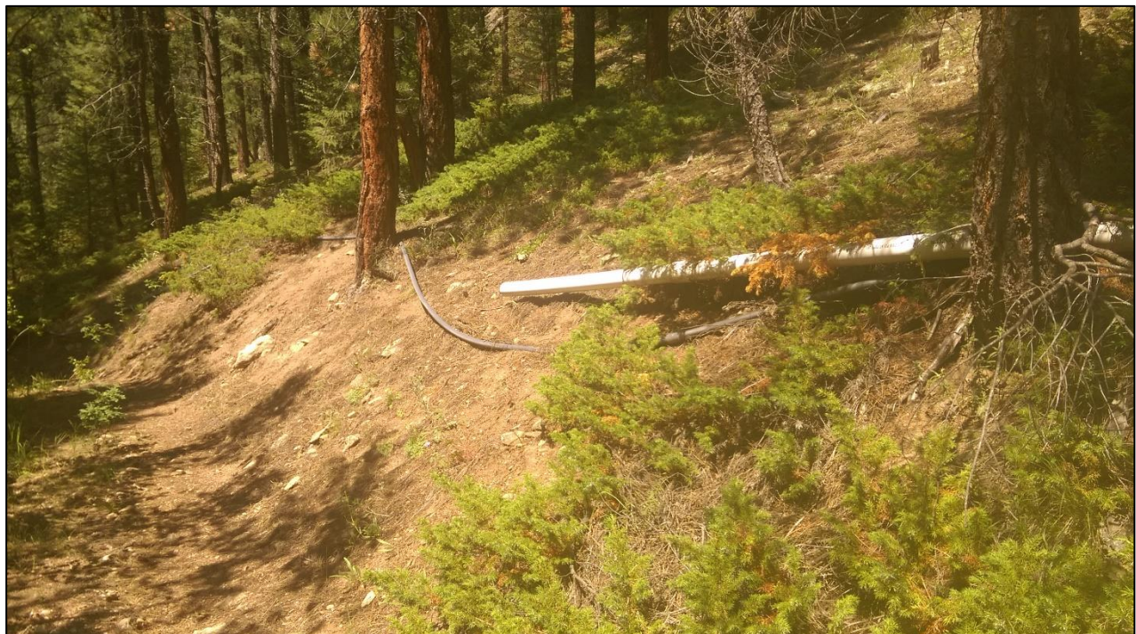
Photo 8. View looking downhill along trail following Lick Skillet Gulch, showing two existing pipelines present along edge of trail. According to Mr. Steen, PVC pipe was installed by him when mill was first constructed in 1980's, and smaller black HDPE pipe was installed by previous operator in 1990's. Note PVC pipe disconnected.
