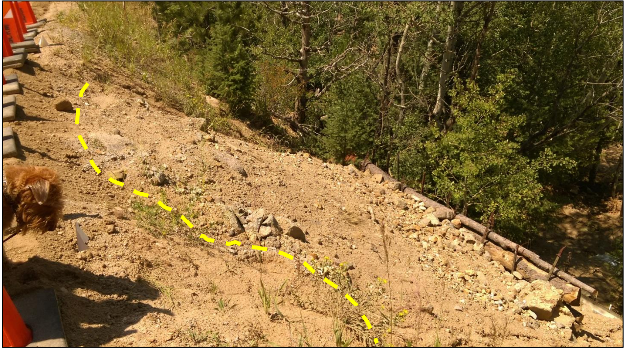
Photo 3. View looking down from northern edge of Sunshine Canyon Drive at Times Mine subsidence area. Approximate edge of subsidence feature (not visible due to fill placement) is indicated with a yellow dashed line.
