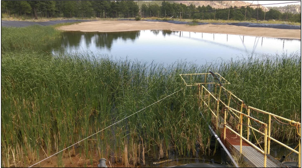
Photo 22. View looking northeast across lined tailings impoundment located east of mill building. Note water and cattails present in western portion of impoundment.
