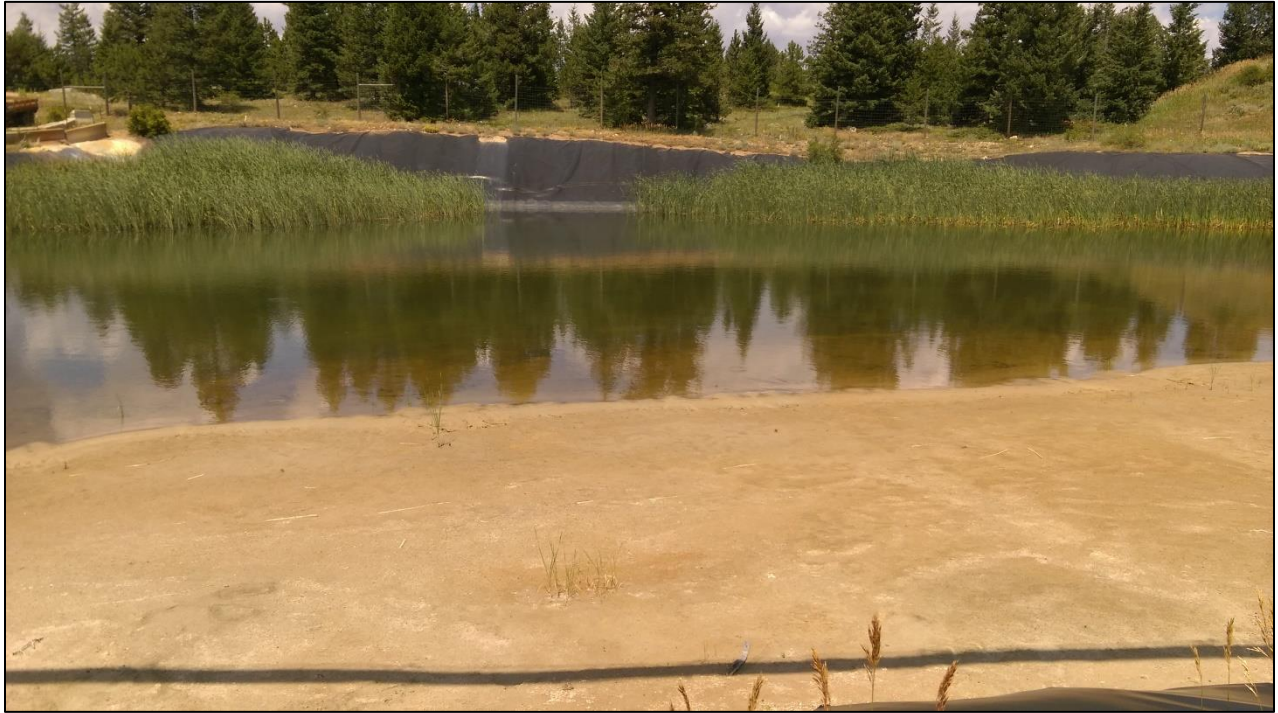
Photo 24. View looking north across lined tailings impoundment. Note available freeboard along northern edge exceeds the required two feet. It should be noted, the northern edge of the impoundment appears to be approximately 2 feet higher in elevation than the southern edge of the impoundment.
