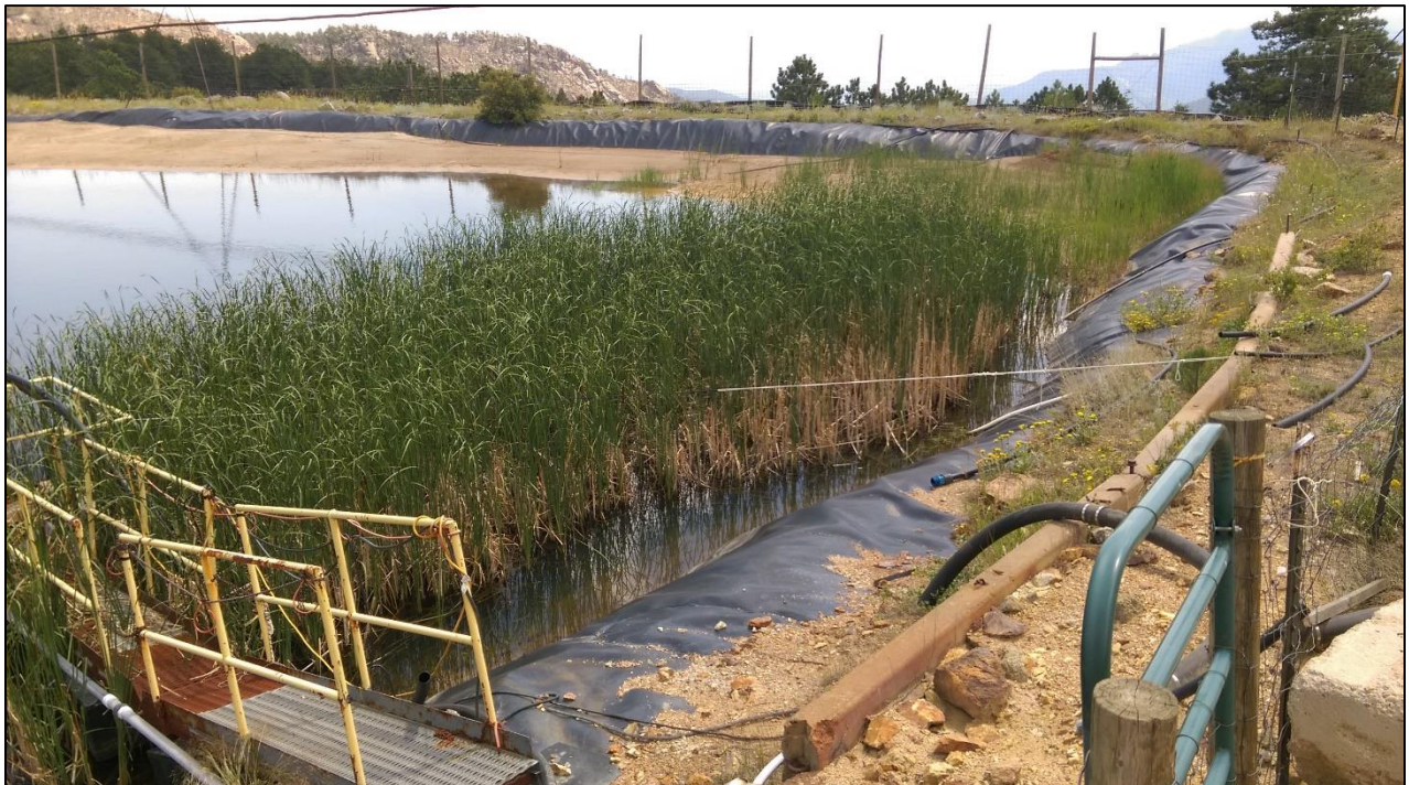
Photo 23. View looking across western edge of lined tailings impoundment. Note water and cattails present in this portion of the impoundment. Also note available freeboard along western edge meets or exceeds the required two feet.
