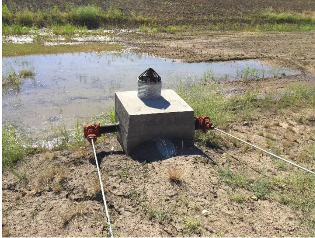
Photo 3 – Pond NHN-002 Primary Spillway
