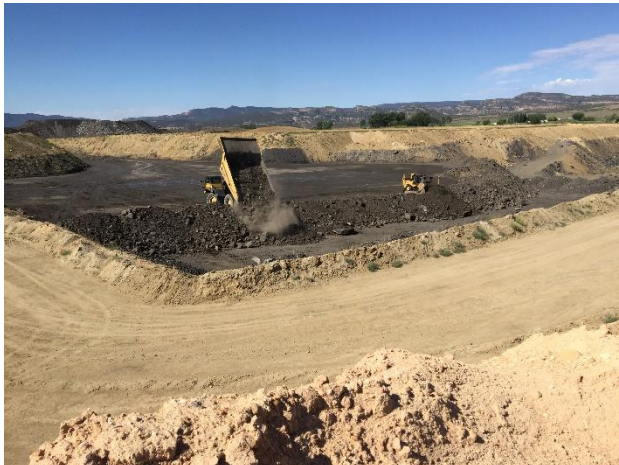
Photo 1 – Backfilling Main Pit Area
