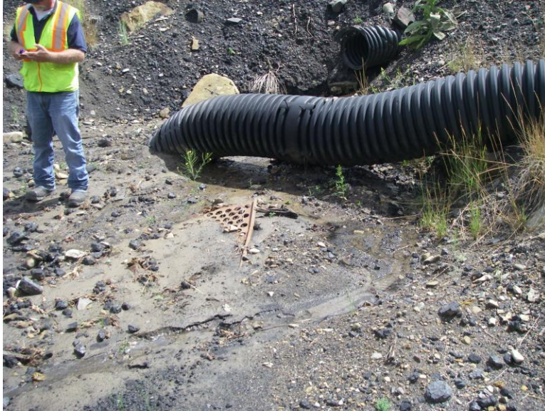
Broken pipe at King I (Reach 3)
