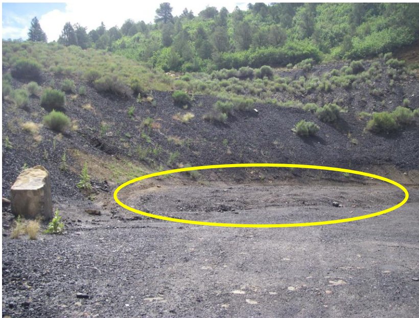
Lower part of Refuse Pile face where the slope is being flattened (recently graded and compacted material within oval)
