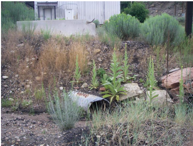
Clogged culvert at King I (lower end of Reach 7)
