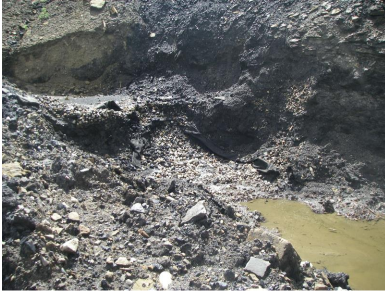
End of underdrain that needs to be extended as slope is extended away from Refuse Pile
