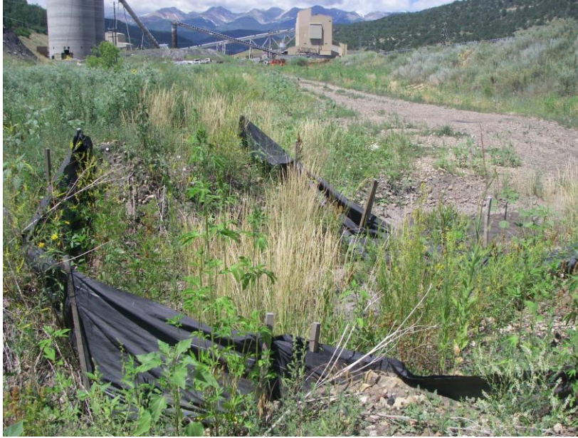
Silt fence below SAE by Pond 007A
